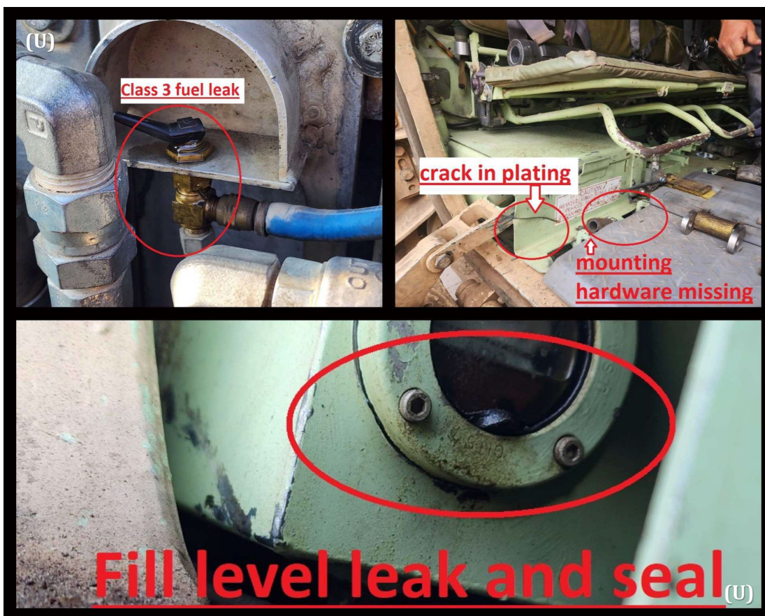
(U) Figure 3. Faults Found During Joint Technical Inspections, Pictures Provided to the DoD OIG in January 2025
