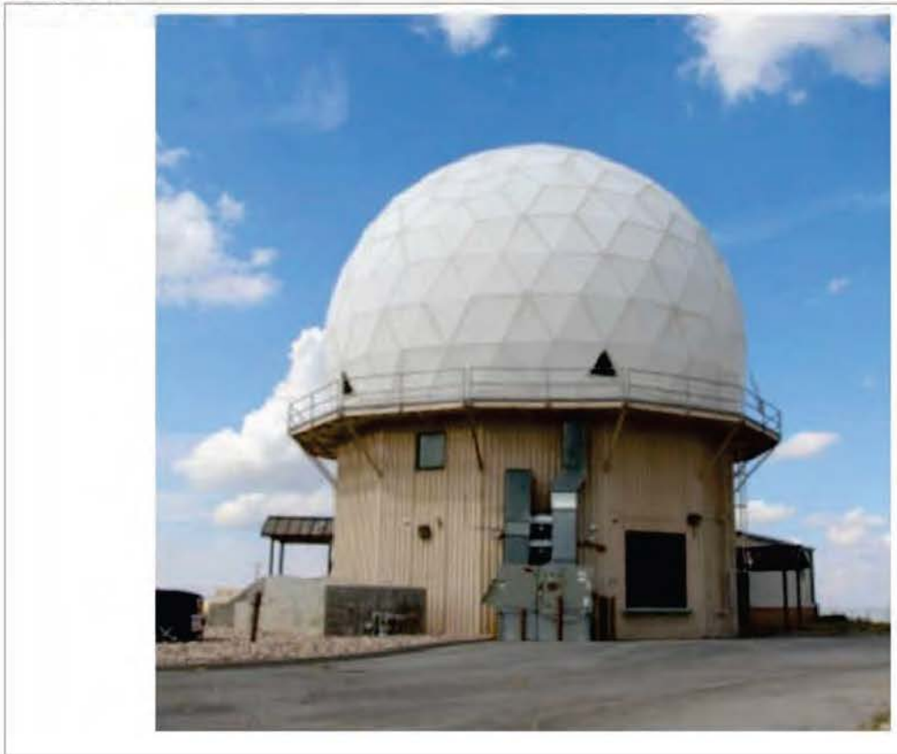
(U) Figure 4. Outside View of the FPS-117 Engineering Facility Radar at Hill Air Force Base, Utah
