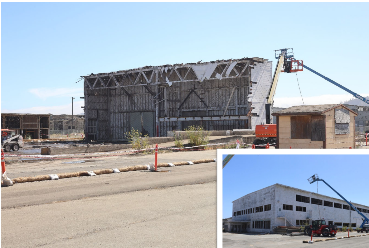
Bldg 401 – Thursday, 09-July-2026: 95% demolished. Concrete Slab still in place.
