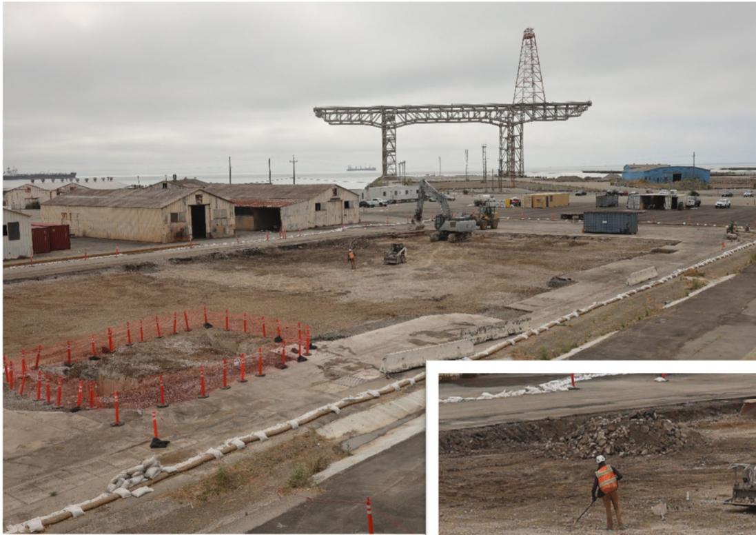
Bldg 351: 06-July-2026: 99.9 % of debris removed
