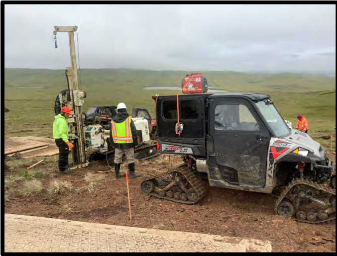
Drilling rig and supporting UTV
