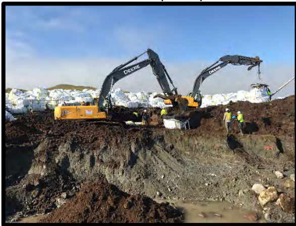
Excavating soil and filling bulk bags
