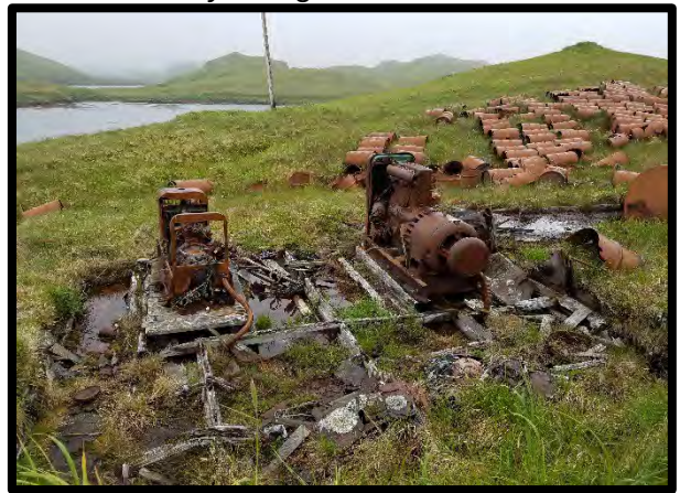
Generators and drums before removal action
