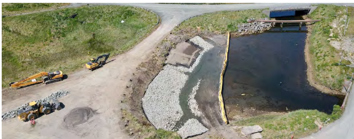
Photo of Oleophilic Bio-Barrier during construction on 11 July 2022
