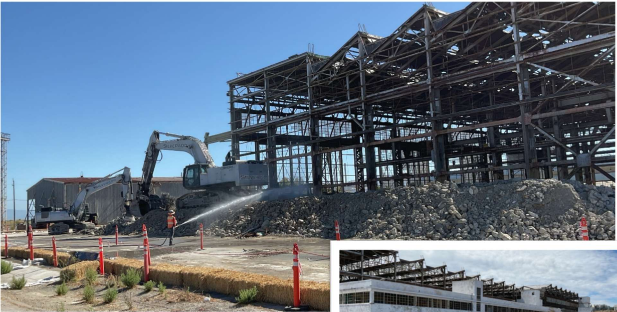
Bldg 411 – Monday, 03-August-2026: Processing debris and material from the South Admin building.
