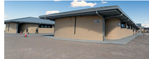
3D Printed Barracks – Fort Bliss, TX
