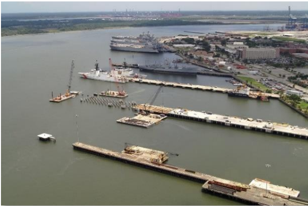
Coast Guard infrastructure is critical to the logistical support required for mission execution and success. (Base Charleston)
