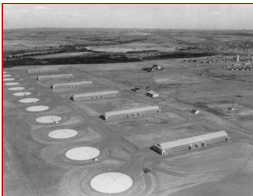
An aerial view of the six Snark assembly and checkout buildings at Presque Isle AFB, Maine. In front of each building are two circular launch pads
