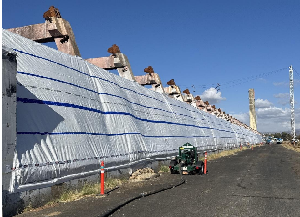
Photo 6 – East side CU construction to support debris removal and prevent fugitive dust.
