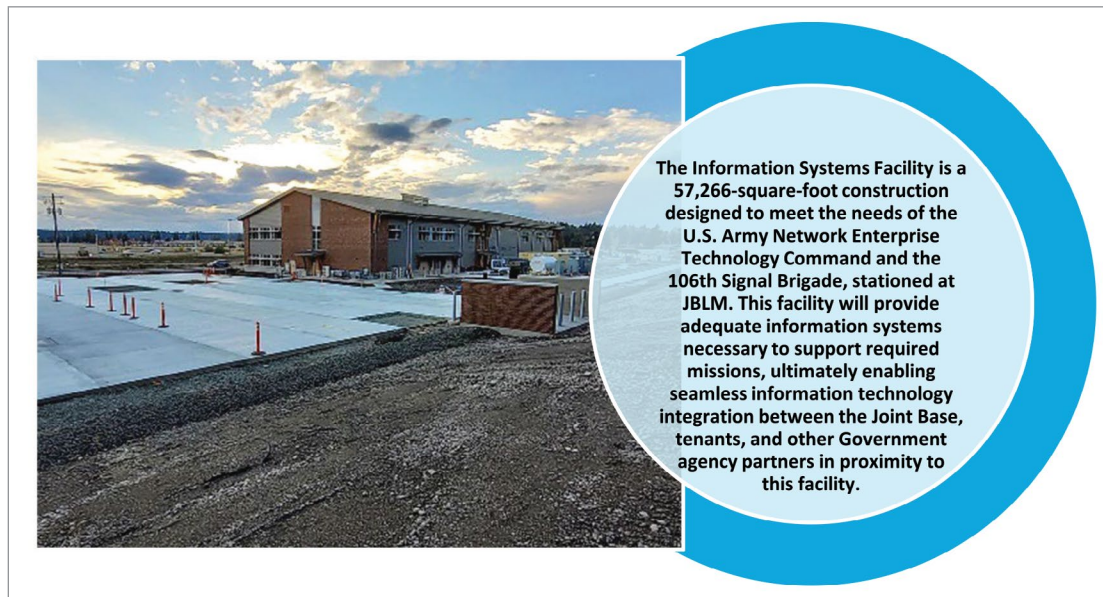
Figure 15. Information Systems Facility at JBLM
