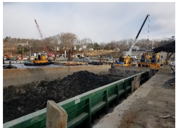
Sediment dewatering; awaiting transport offsite
