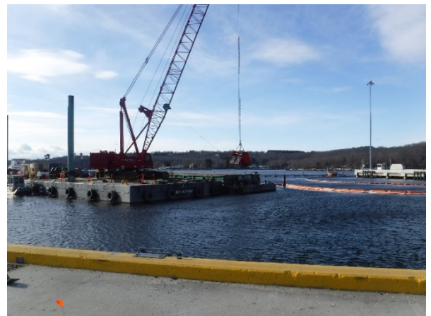
Dredge barge in dredge area with crane and environmental bucket
