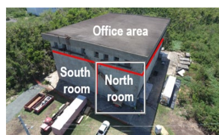
NAVAL ACTIVITY PUERTO RICO FORMERLY NAVAL STATION ROOSEVELT ROADS
