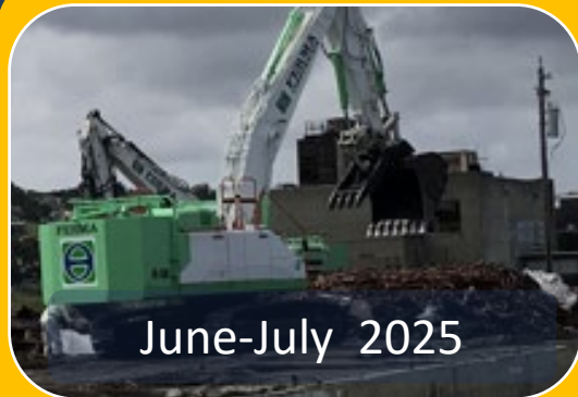
Excavate soil and take confirmation samples
