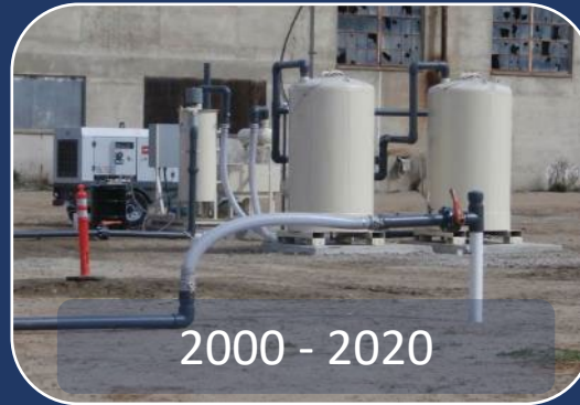
Equipment used to extract soil vapors; additional cleanup needed
