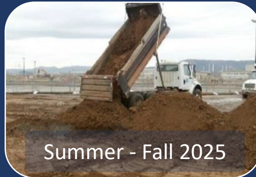
Backfill excavation site with clean soil
