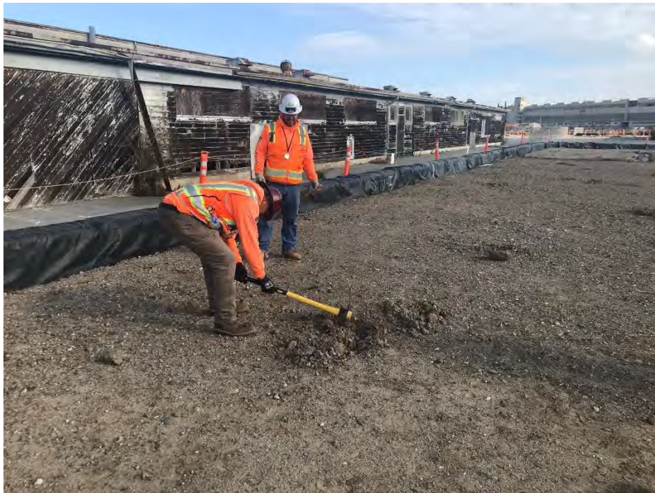
Figure 2 – HPT loosening the soil around the LLRO with a pickaxe
