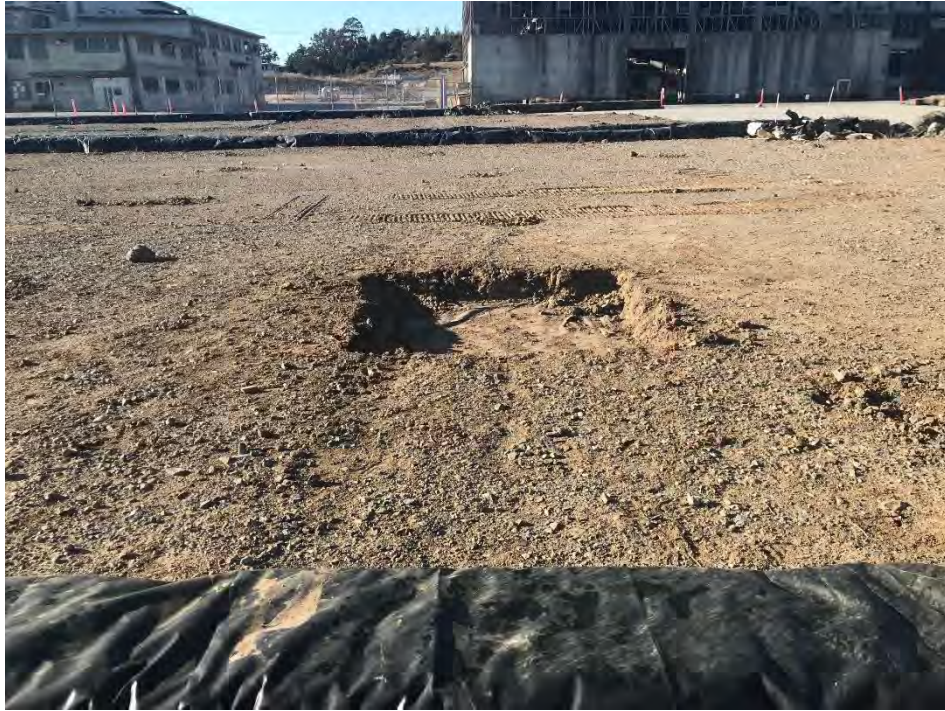
Figure 1 – A 5 ft x 5 ft area of soil was excavated around the LLRO location
