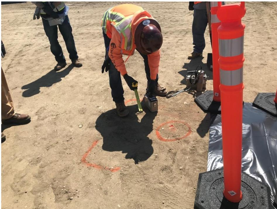
Figure 3 – Exposure rate measurement 30 cm away from the LLRO location
