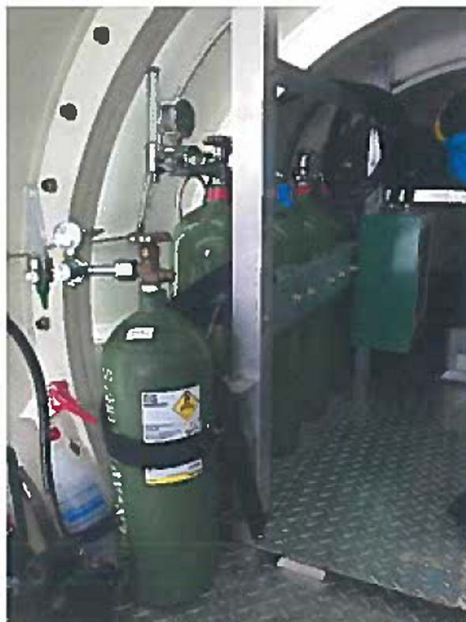
Image showing Starboard O 2 system.
