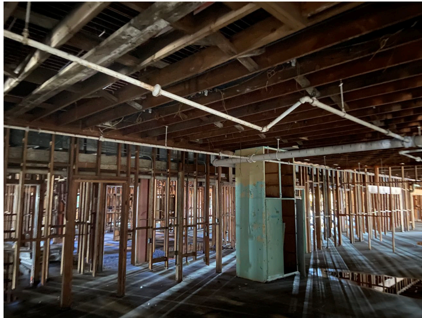
Figure 5: Building 351A Interior
