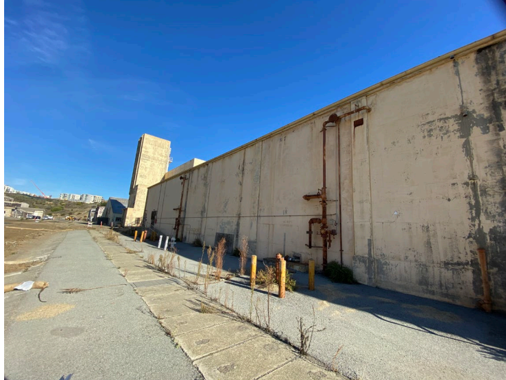
Figure 4: Building 351A Exterior
