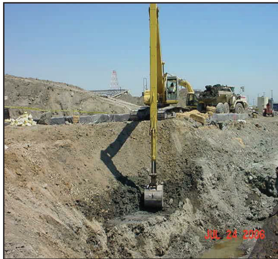
Excavation up to 20 feet
