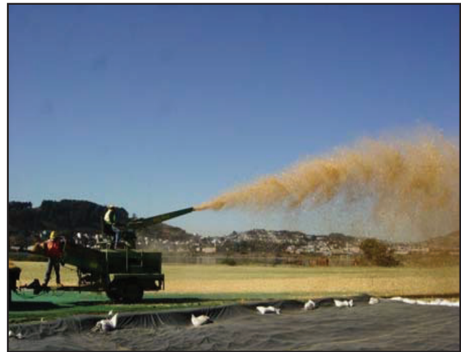
Hydroseeding and Spreading Hay for Protection
