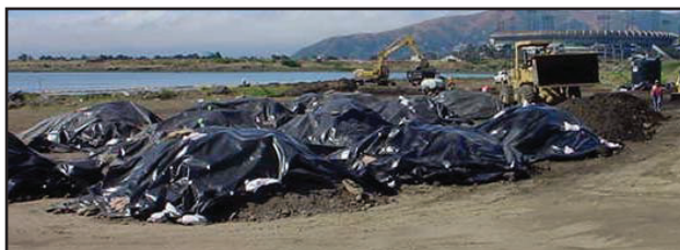
Soil Excavated for Off-Site Disposal
