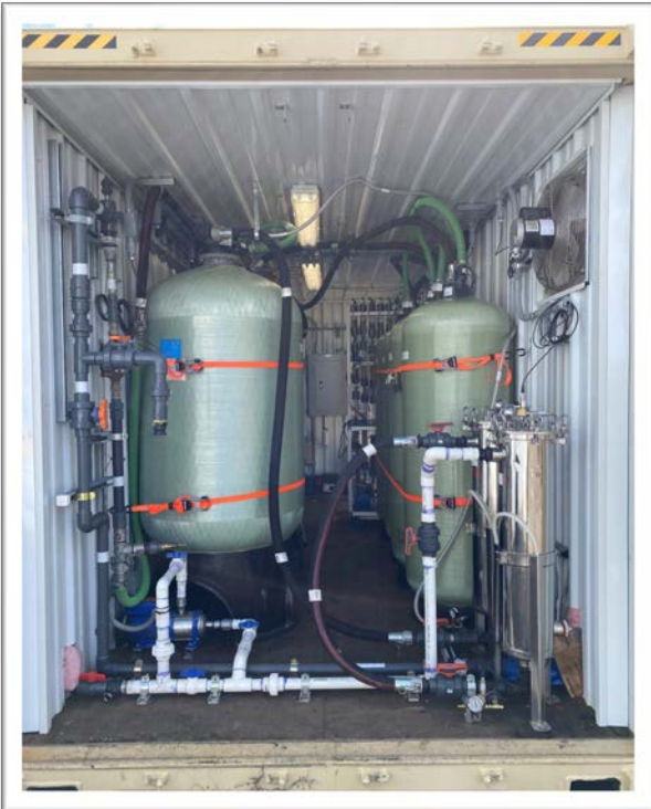
Hangar 680 PFAS Pilot Test Treatment System Source: Tetra Tech
