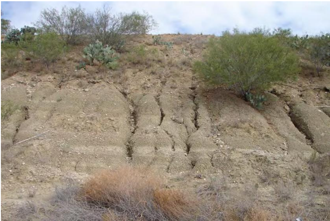
Casa Blanca Dam erosion on downstream slope. (14 September 2006 Site Visit)
