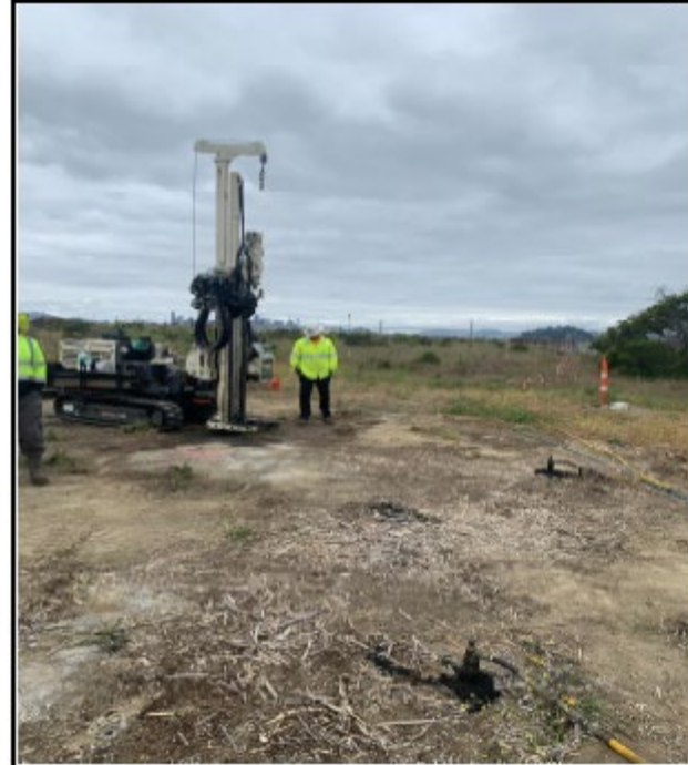
Injection in process
