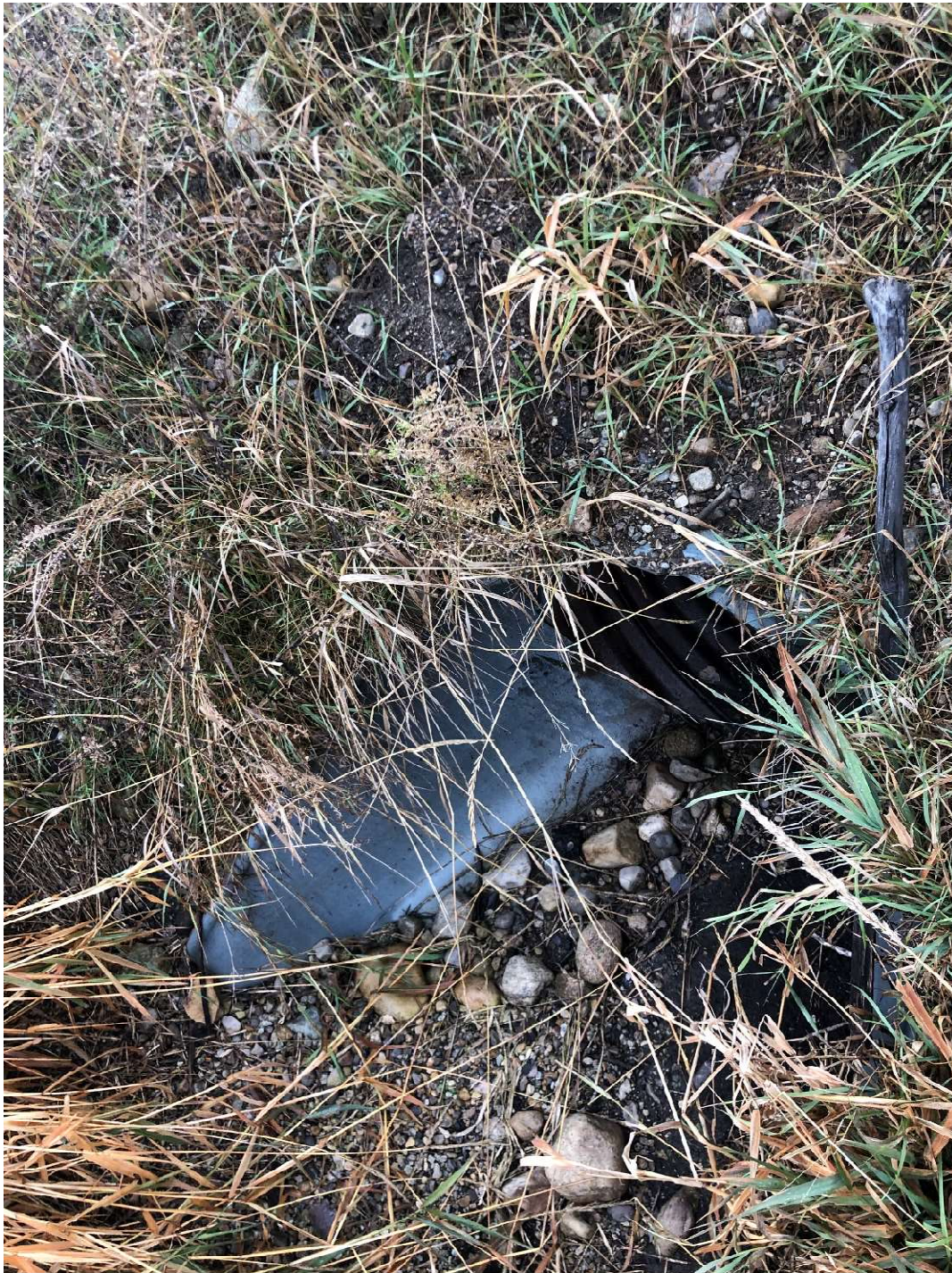
Photo 6. Culvert on East side of Highway 33. Taken from Photo Point 2.
