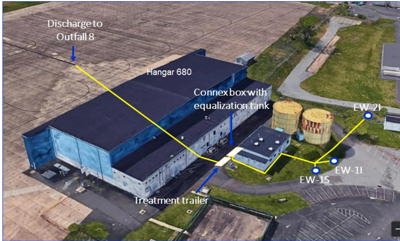
Location of Hangar 680 treatment system
