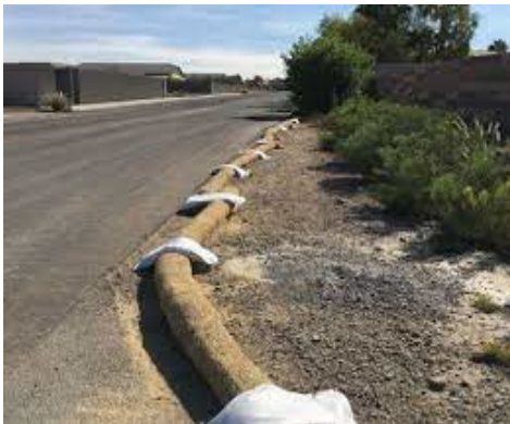
Fiber rolls are used as sediment control for stormwater BMPs
