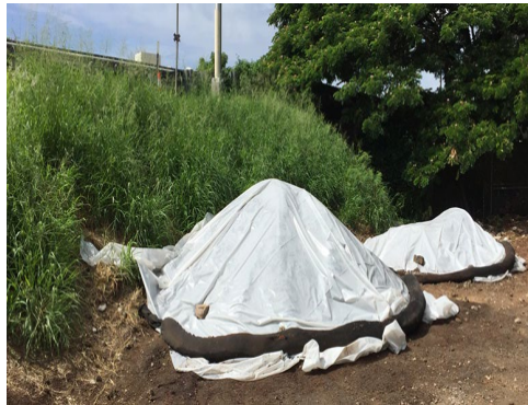
Stockpile protection includes plastic tarps and fiber rolls
