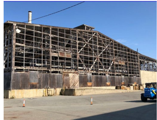
Demolition of Building 123 allows access to remove contaminants from underlying soil
