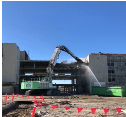
Modified Excavators with on-board water and high-pressure water nozzles minimize dust
