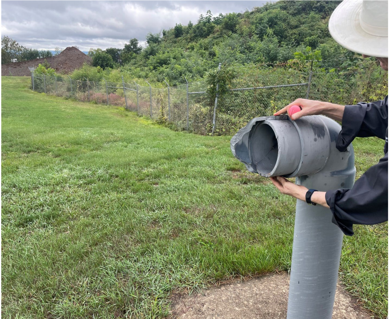
Photo S2: Landfill vent has been damaged from being struck by golf balls on the driving range. The perpendicular portion of the vent is still sufficiently shielded from precipitation and foreign debris.
