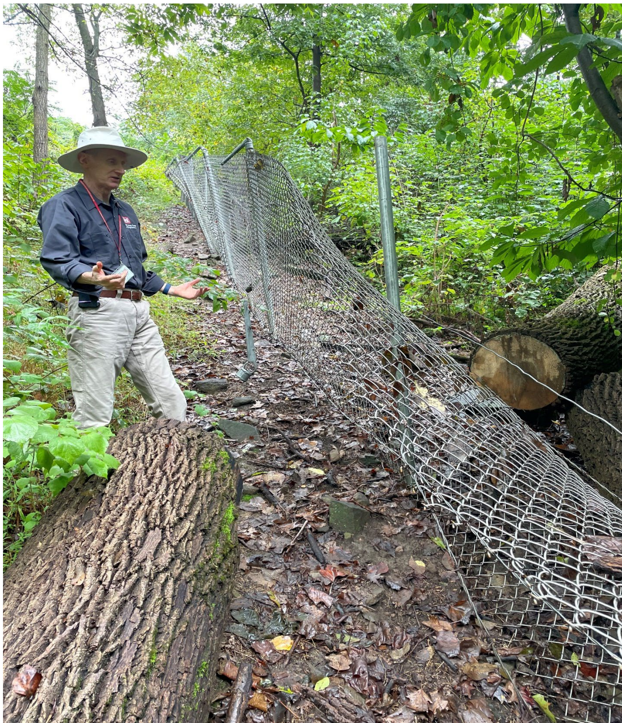
Photo S10: Perimeter fencing needs to be repaired from fallen trees.
