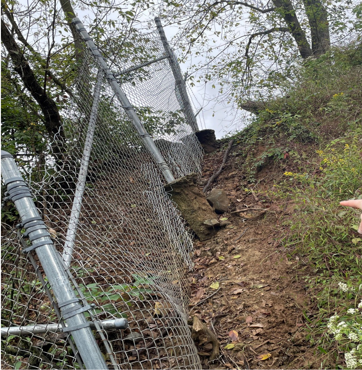
Photo S4: The perimeter fence is intact, but erosion has exposed the foundation of the fence post.
