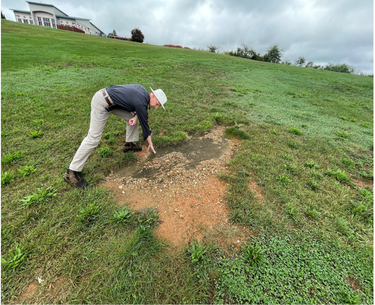
Photo S1: The soil of the landfill cap has eroded in various places, exposing the liner in this location. This patch measures approximately 4.5 by 7.5 feet.
