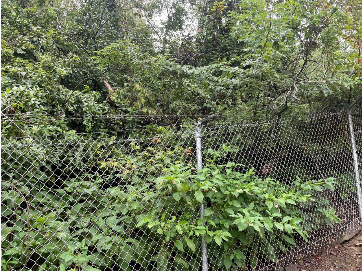
Photo S6: Perimeter fence barbedwire intact but needs to be repaired. Also, vegetation needs to be trimmed along the perimeter fence.
