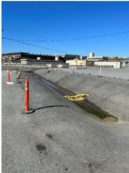
Parcel D-1 Photograph 4: Drainage swale adjacent to Parcel G. Facing southwest.
