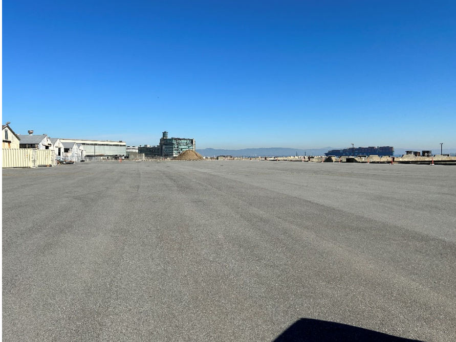
Parcel D-1 Photograph 1: Asphalt pavement cover adjacent to Parcel G. Facing northeast.
