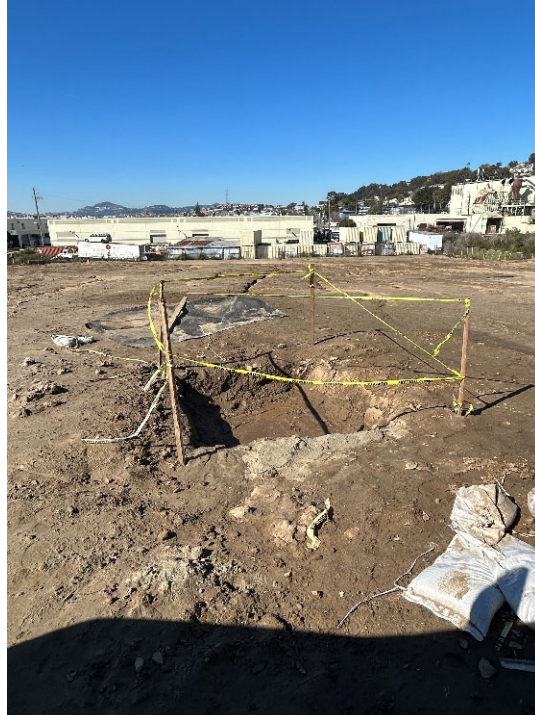
Parcel E2 Photograph 11: Small excavated area with sandbags. Facing southwest. Photographed by: Marcella Navas/CH2M, 2/9/2023
