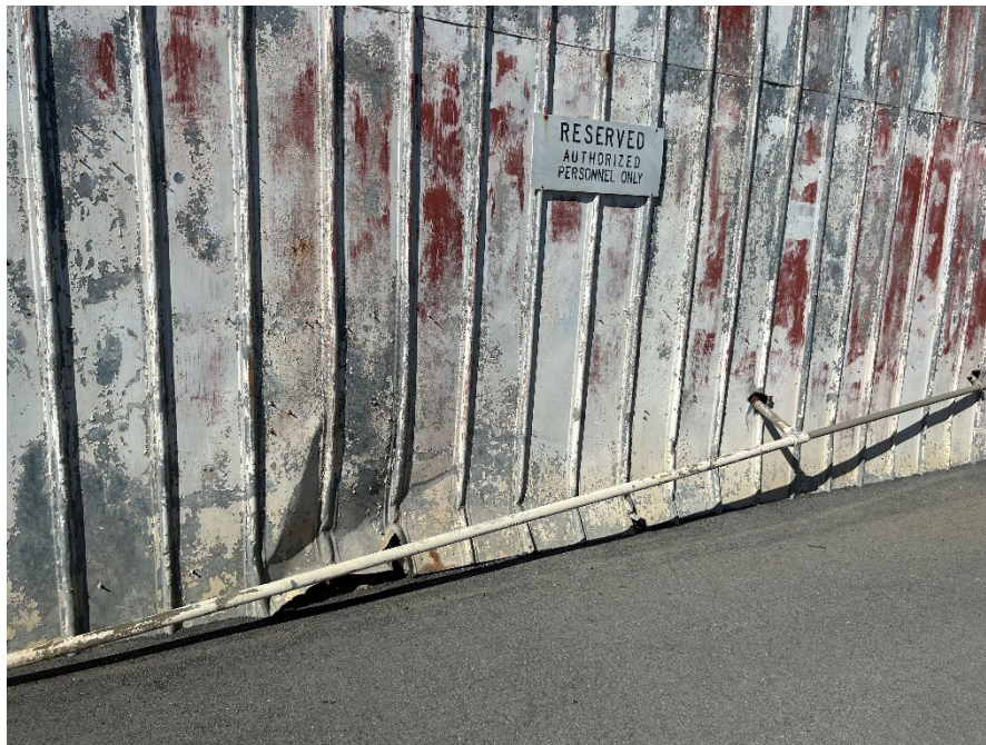
Parcel D-1 Photograph 16: Building 526 foundation. Facing southeast. Photographed by: Marcella Navas/CH2M, 2/9/2023
