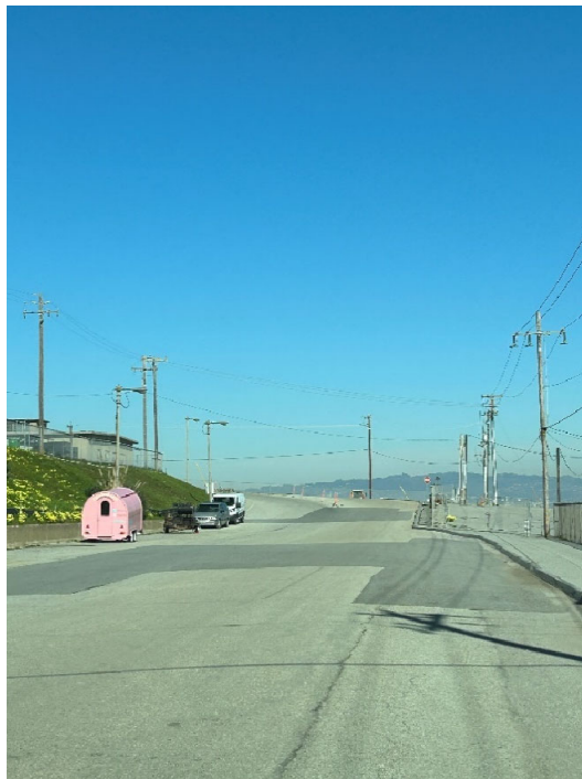
Parcel UC-2 Photograph 3: Asphalt pavement cover along Fisher Avenue. Facing northeast.
