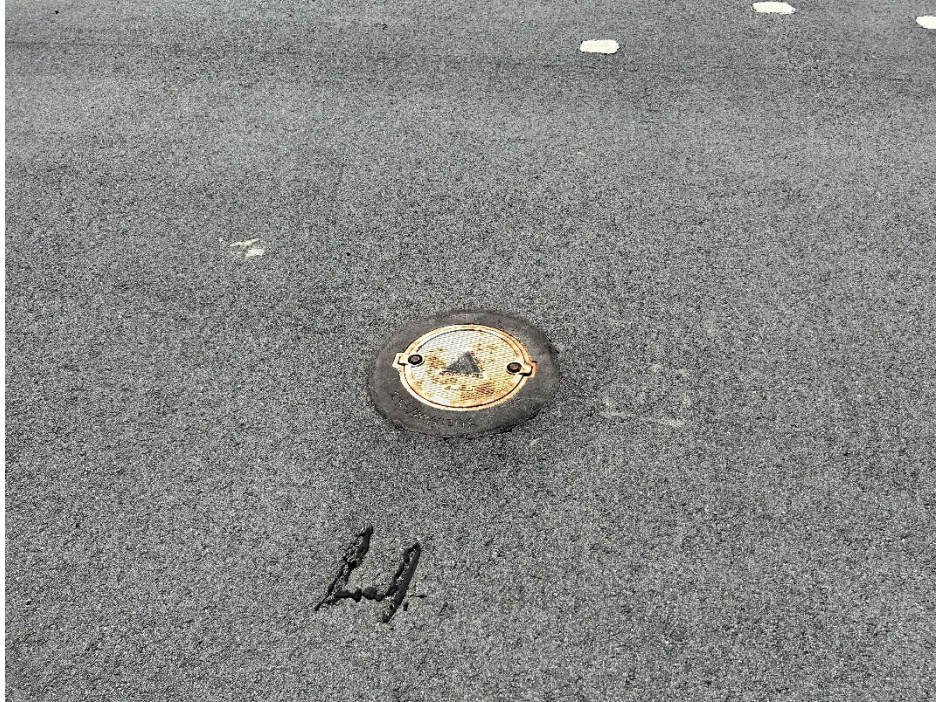
Parcel D-1 Photograph 19: Monitoring well completion and repaired boreholes east of Building 523. Facing southwest.
