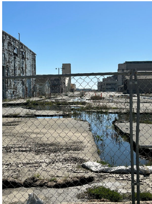
Parcel G Photograph 16: Trenching between Building 402 and 302 within Parcel G from UC-1. Facing southeast. Photographed by: Marcella Navas/CH2M, 2/9/2023
