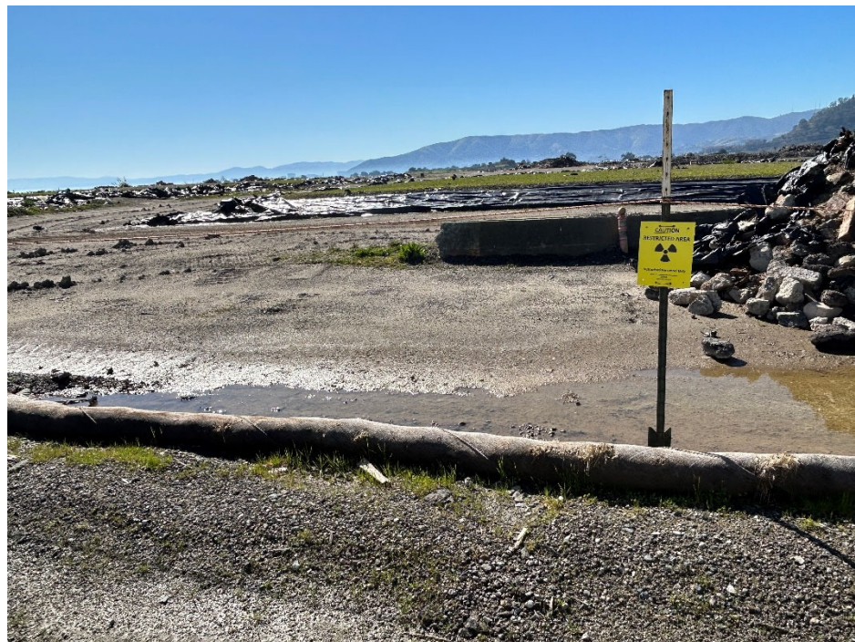
Parcel E Photograph 6: Restricted Area signage, stockpile, and best management practice on the corner of 6th Avenue and J Street. Facing southeast.
