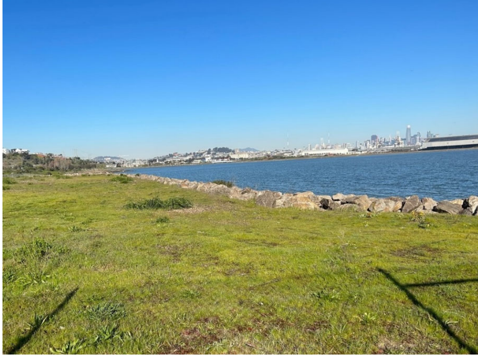
IR-07/18 Photograph 1: Soil cover near revetment crest. Facing northwest. Photographed by: Marcella Navas/CH2M, 2/9/2023
