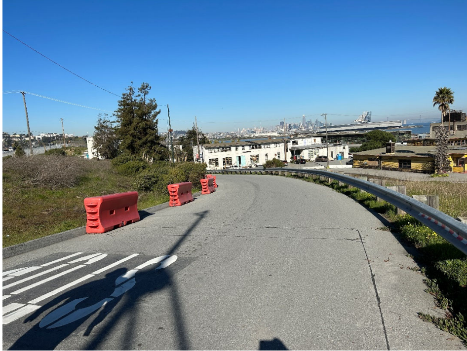
Parcel B-1 Photograph 11: Asphalt cover southwest of Building 113. Facing northwest. Photographed by: Marcella Navas/CH2M, 2/9/2023
