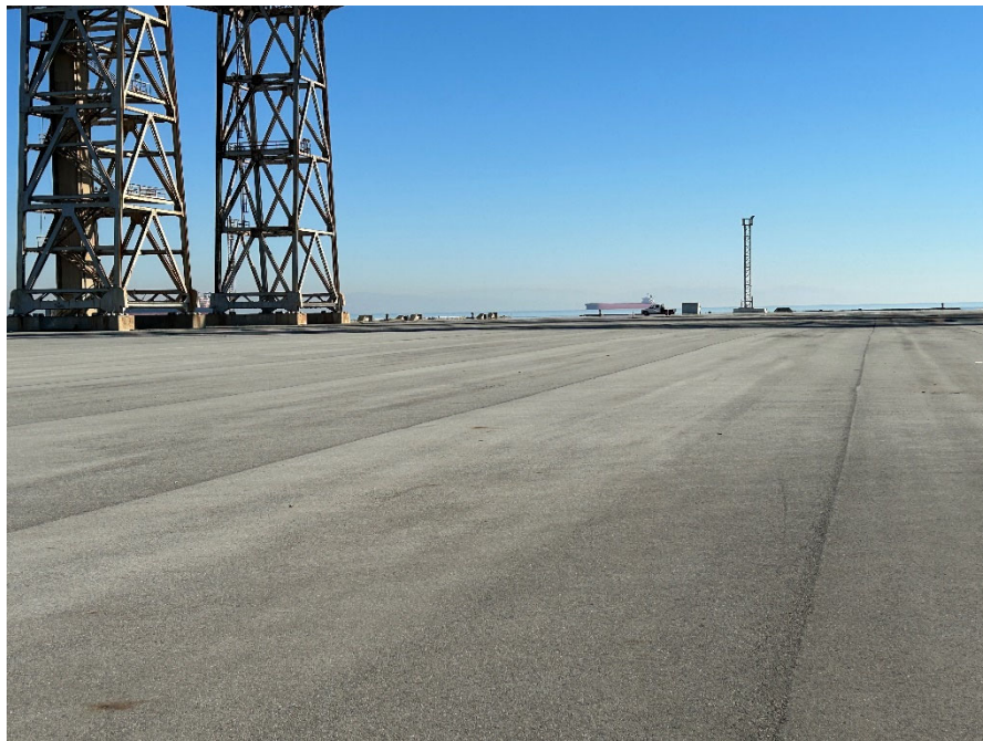
Parcel D-1 Photograph 12: Asphalt pavement cover between Buildings 381 and 383. Facing northeast.
