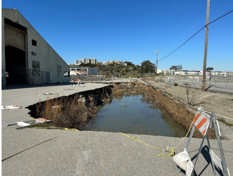
Parcel G Photograph 5: Trenching east of Building 366. Facing northeast.
