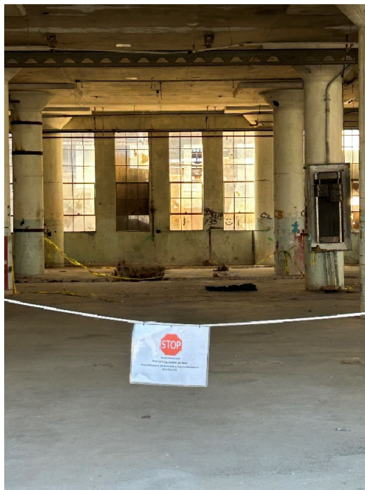
Parcel G Photograph 8: Warning sign outside of Building 351. Facing southwest.
