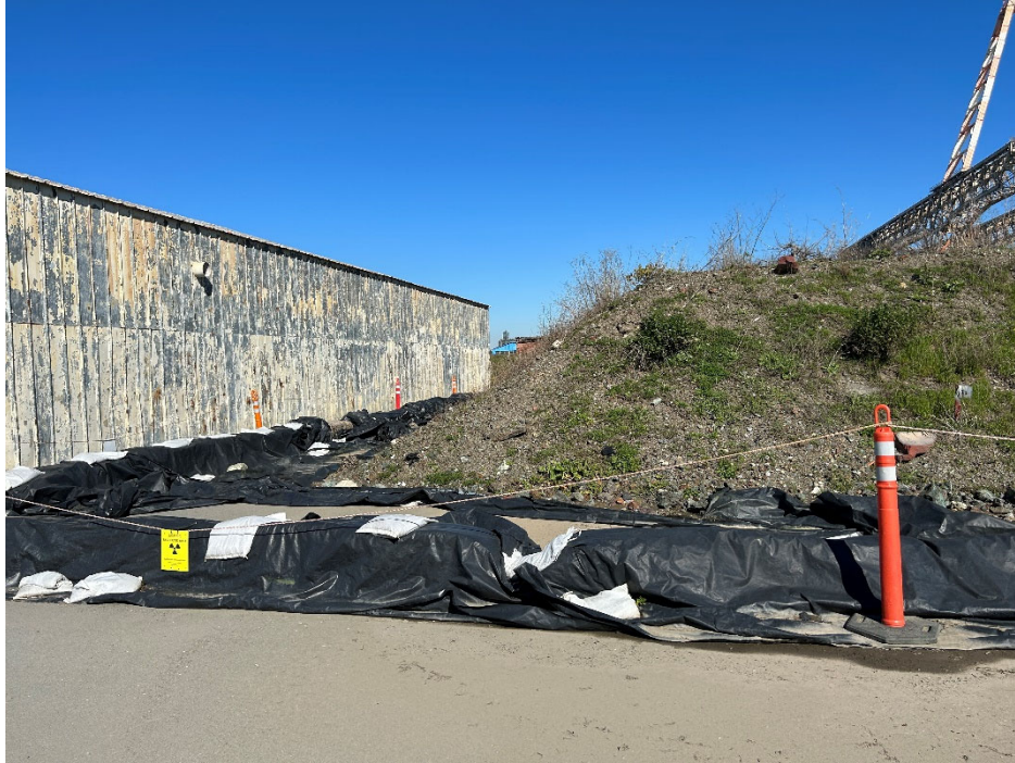
Parcel D-1 Photograph 15: Stockpile east of Building 525 within secondary containment and signage. Facing northeast. Photographed by: Marcella Navas/CH2M, 2/9/2023
