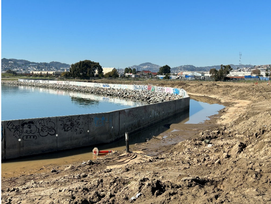
Parcel E-2 Photograph 7: Accumulated water and monitoring well adjacent to shoreline revetment and seawall. Facing southwest.
