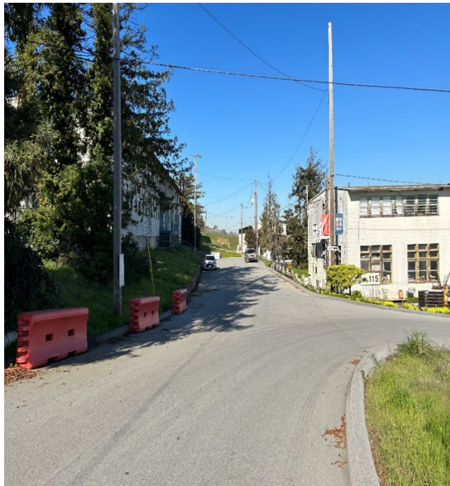
Parcel B-1 Photograph 12: Driveway northeast of Buildings 103 and 117. Facing northwest. Photographed by: Marcella Navas/CH2M, 2/9/2023
