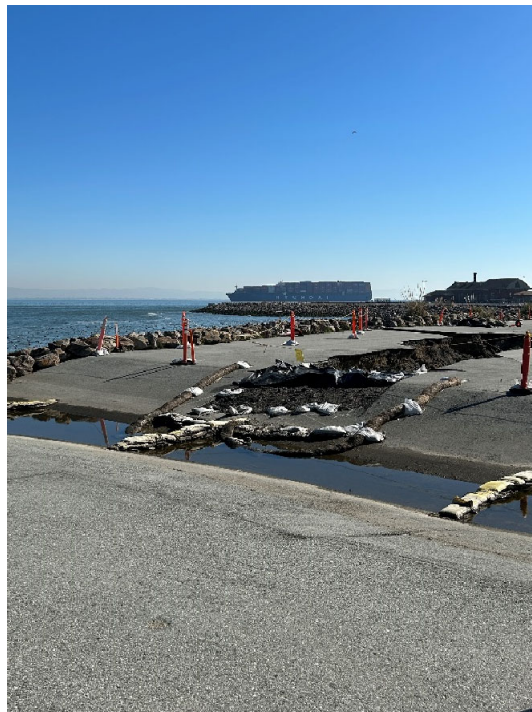
Parcel B-2 Photograph 6: Trenching east of Building 130. Facing northeast.
