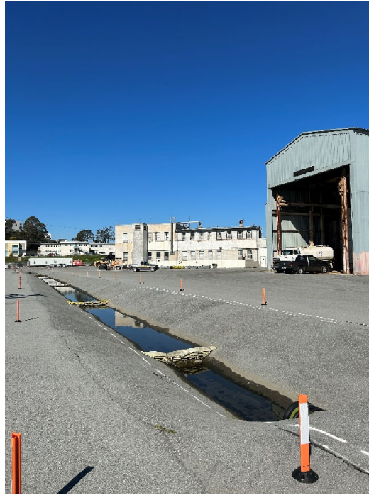
Parcel C Photograph 15: Paved drainage swale southwest of Building 230. Facing northwest.
