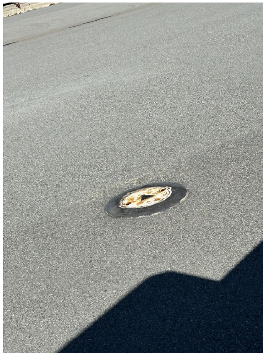
Parcel C Photograph 18: Monitoring well south of Building 271 along Nimitz Avenue. Facing northwest.
