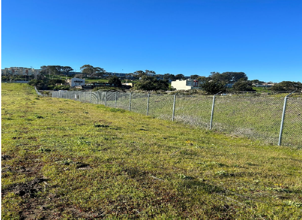
IR-07/18 Photograph 15: Chain-link fence along non-Navy property. Facing southwest.
