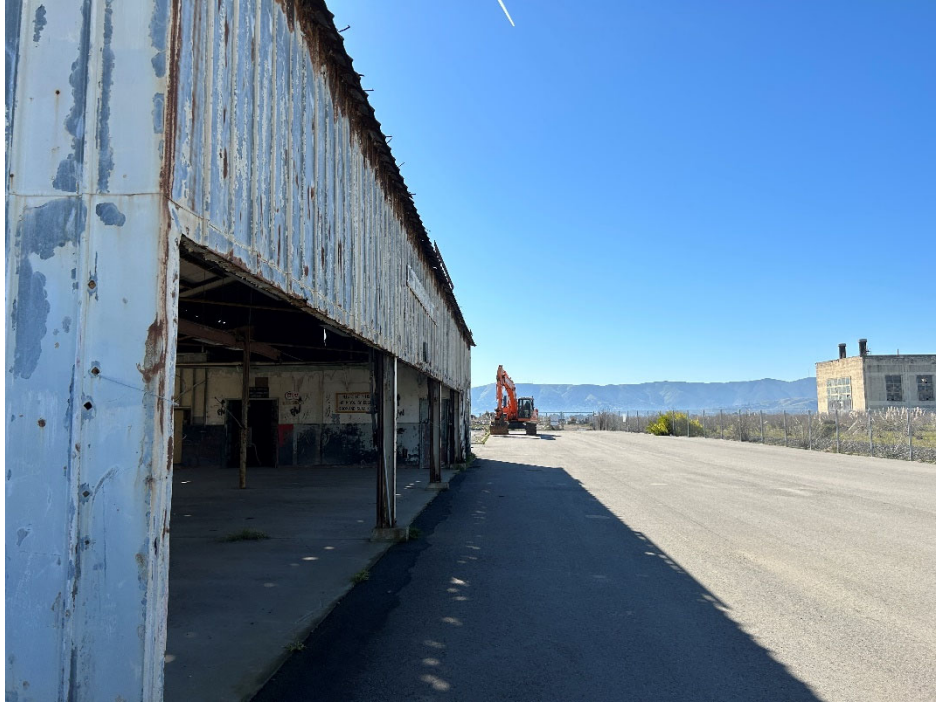
Parcel D-1 Photograph 13: Asphalt pavement cover adjacent to Building 530. Facing southwest.
