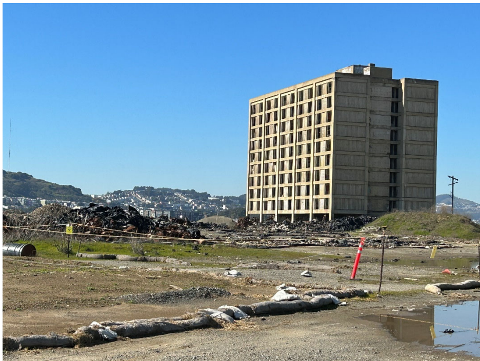
Parcel E Photograph 10: Building 521 with cordoned work area and warning signs. Facing southwest.
