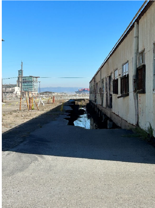
Parcel G Photograph 7: Trenching northwest of Building 363. Facing north.
