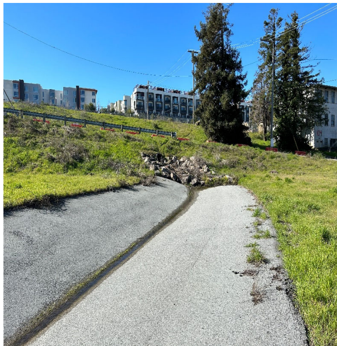
Parcel B-1 Photograph 14: Drainage swale in asphalt pavement cover southwest of Building 120. Facing southwest.
