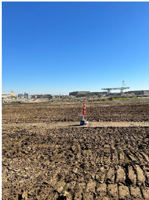
Parcel E-2 Photograph 4: Graded area with marked monitoring point. Facing southeast.
