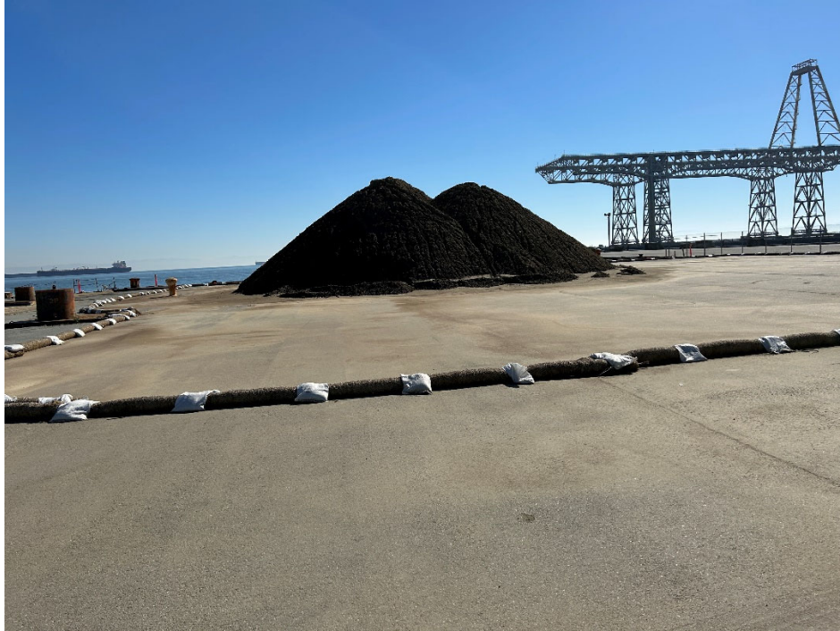
Parcel C Photograph 11: Storage of stockpiles with stormwater management best management practices surrounding and intact. Facing northeast.
