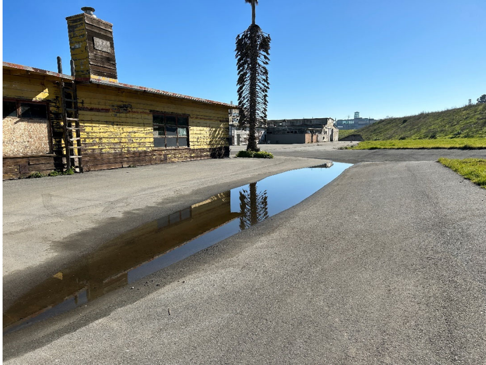
Parcel B-1 Photograph 9: Drainage swale in asphalt pavement cover southwest of Building 120, with small accumulation of water. Facing southeast.
