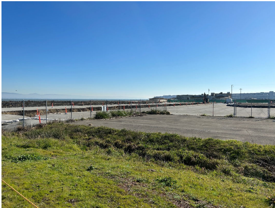
IR-07/18 Photograph 12: Asphalt pavement at bump-out area north of Building 146 and vegetated drainage swale. Facing east.
