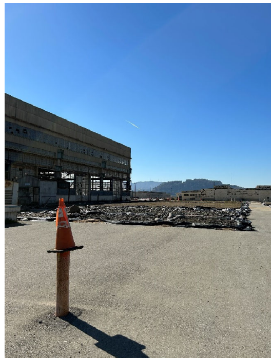
Parcel G Photograph 4: Stormwater best management practice east of Building 418. Facing southeast.
