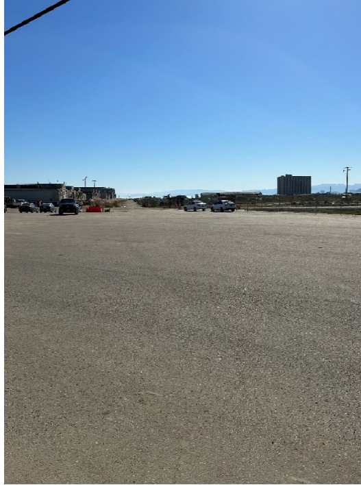
Parcel UC-3 Photograph 7: Asphalt pavement cover between Parcel UC-3 and UC-1. Facing south.
