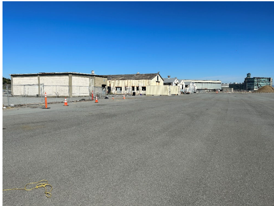
Parcel D-1 Photograph 2: Asphalt pavement cover adjacent to Buildings 306 and 274. Facing northwest.
