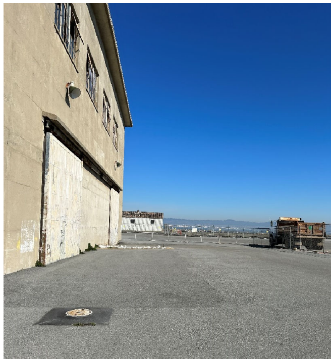
Parcel C Photograph 6: Asphalt pavement cover southeast of Building 134. Facing north.
