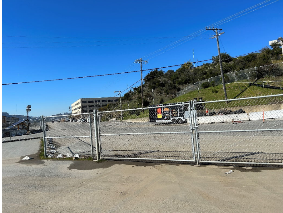
Parcel C Photograph 17: Chain-link fence in between parcel UC-2 along Fischer Avenue. Facing west.
