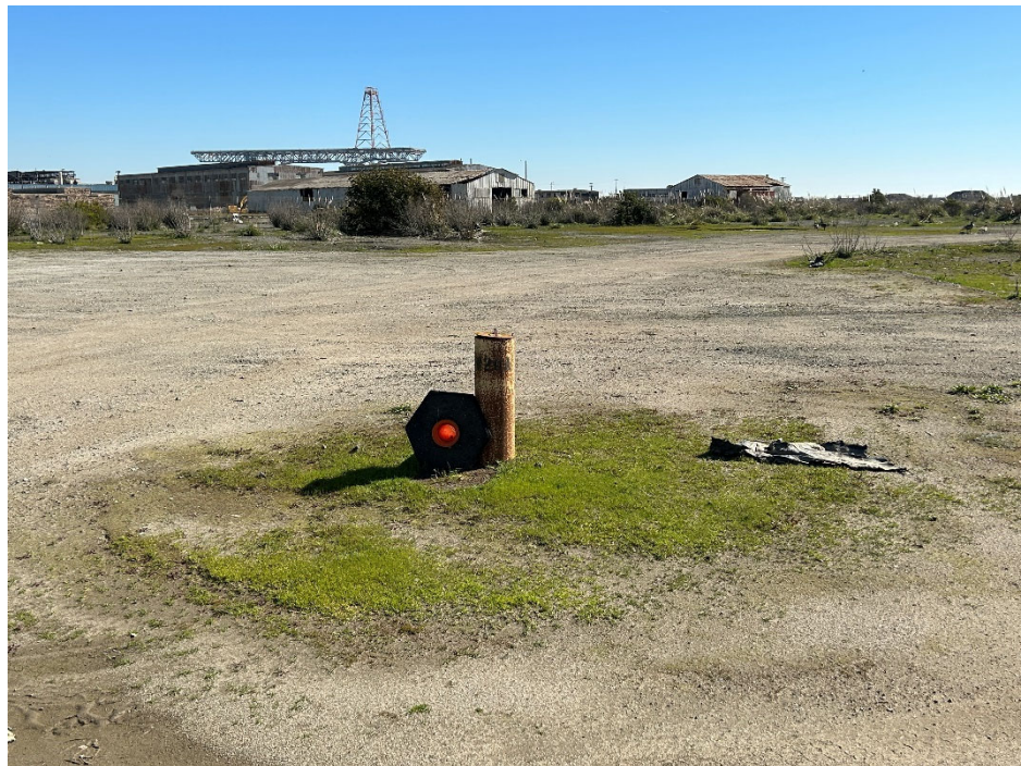
Parcel E Photograph 16: Monitoring well intact and in good condition. Facing northeast. Photographed by: Marcella Navas/CH2M, 2/9/2023
