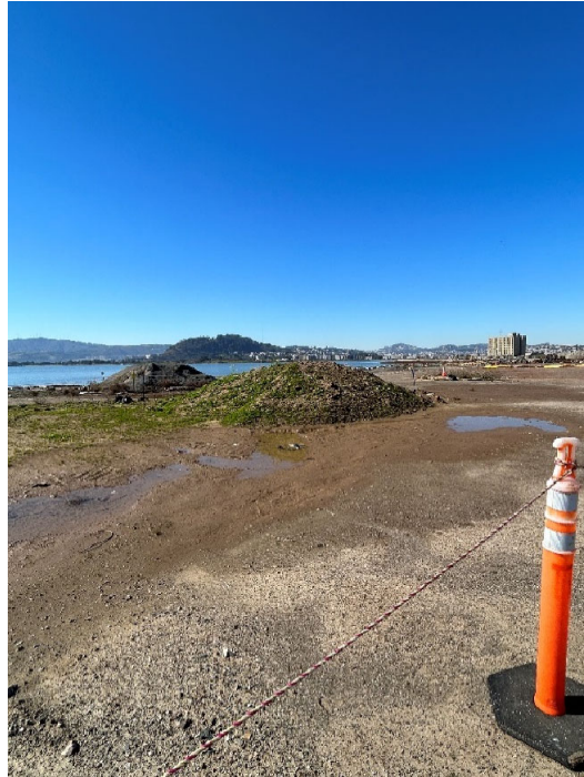
Parcel E Photograph 1: Soil stockpile at the intersection of J and Mahan Street with delineator barricading. Facing southwest.
