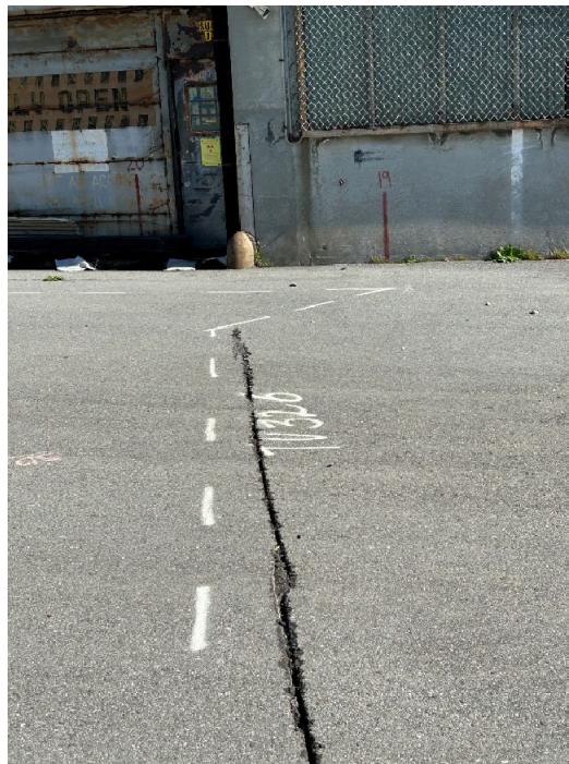
Parcel C Photograph 20: Planned excavation area west of Building 253. Facing east. Photographed by: Marcella Navas/CH2M, 2/9/2023
