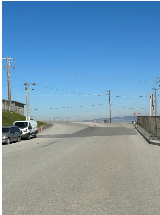
Parcel UC-2 Photograph 1: Asphalt pavement cover along Fisher Avenue. Facing northeast.
