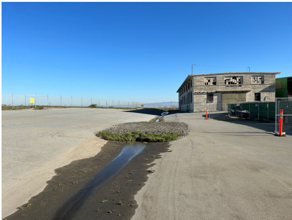
IR-07/18 Photograph 8: Drainage channel with gravel patch southwest of Building 146. Facing northeast.
