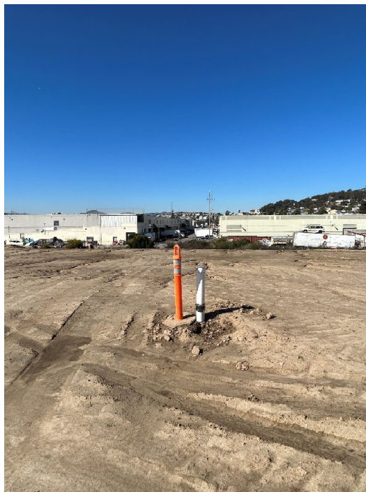
Parcel E-2 Photograph 8: Monitoring well located in soil cover area. Facing southwest.
