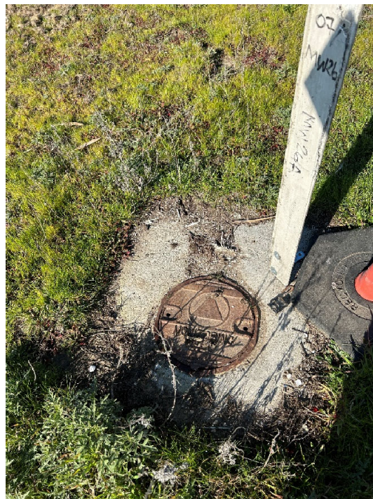
IR-07/18 Photograph 16: Monitoring well southwest of revetment crest. Facing northeast.
