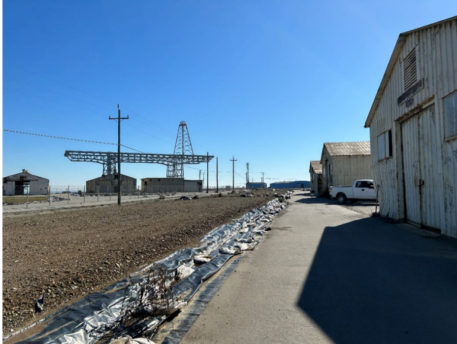
Parcel G Photograph 9: Stormwater best management practice along southeast portion of Parcel G along Buildings 415, 323, and 324. Facing southeast. Photographed by: Marcella Navas/CH2M, 2/9/2023
