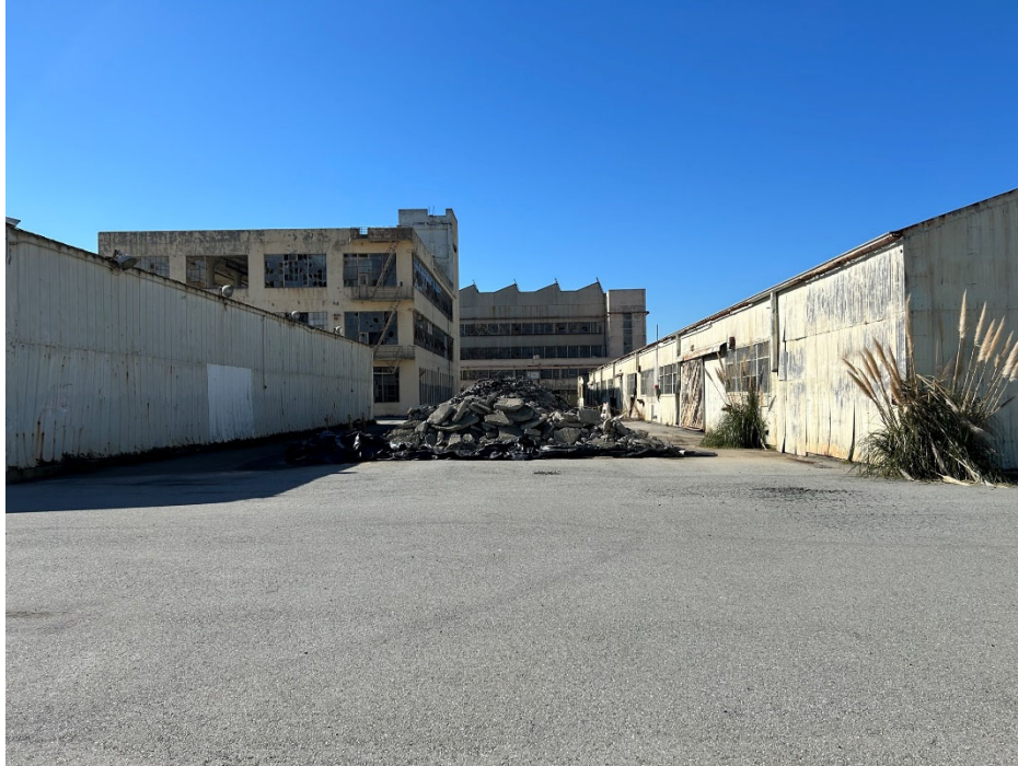
Parcel G Photograph 13: Stockpile between Building 415 and Building 366. Facing west. Photographed by: Marcella Navas/CH2M, 2/9/2023
