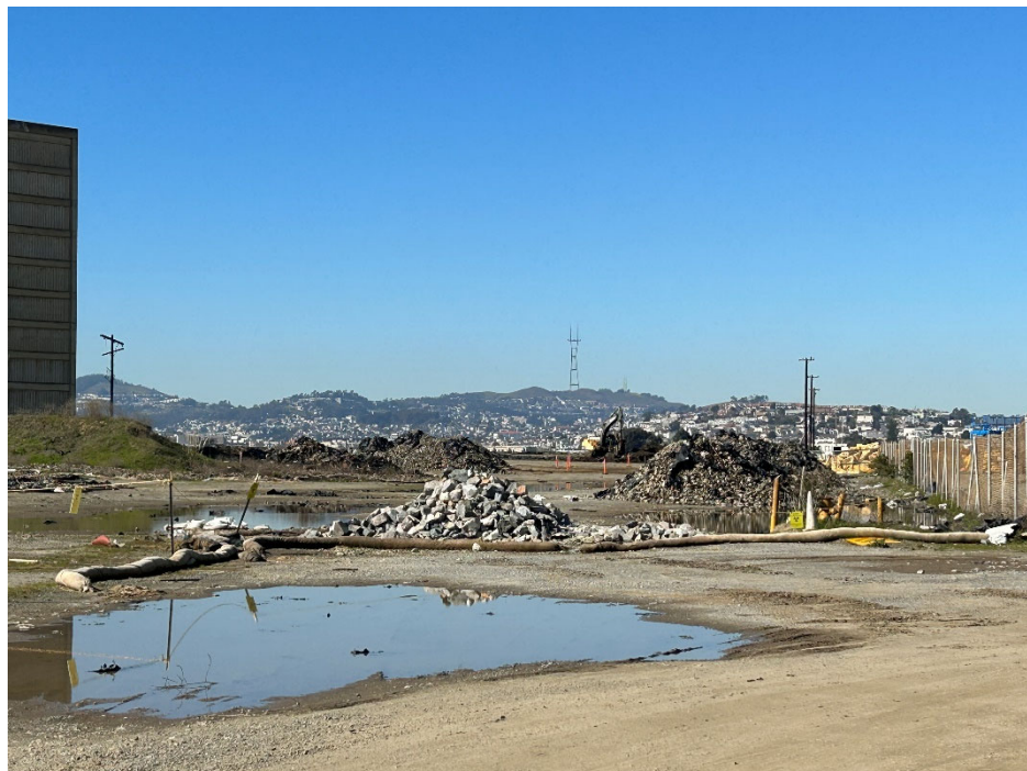
Parcel E Photograph 8: Stockpiles along fence line. Facing southwest.
