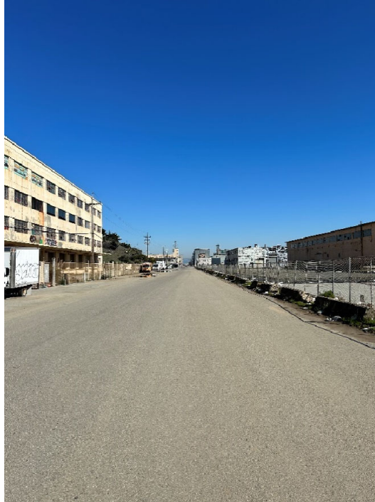
Parcel UC-1 Photograph 3: Asphalt pavement cover along Spear Avenue. Facing northeast.
