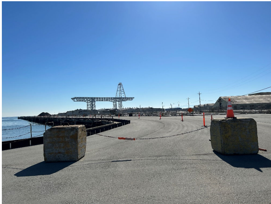
Parcel C Photograph 8: Asphalt pavement cover alongside Parcel G and Parcel U2. Barrier to prevent access. Facing south.
