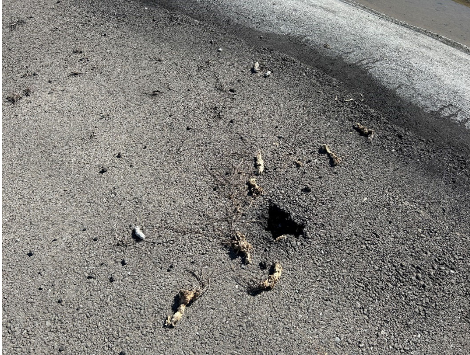
Parcel D1 Photograph 7: Hole and vegetation adjacent to asphalt drainage swale. Facing northwest.
