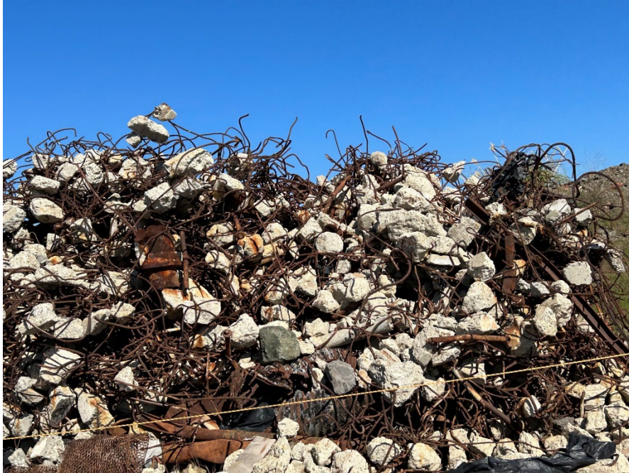
Parcel E Photograph 3: Construction debris. Facing southeast. Photographed by: Marcella Navas/CH2M, 2/9/2023
