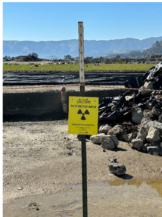
Parcel E Photograph 18: Caution sign around active work. Facing southeast.
