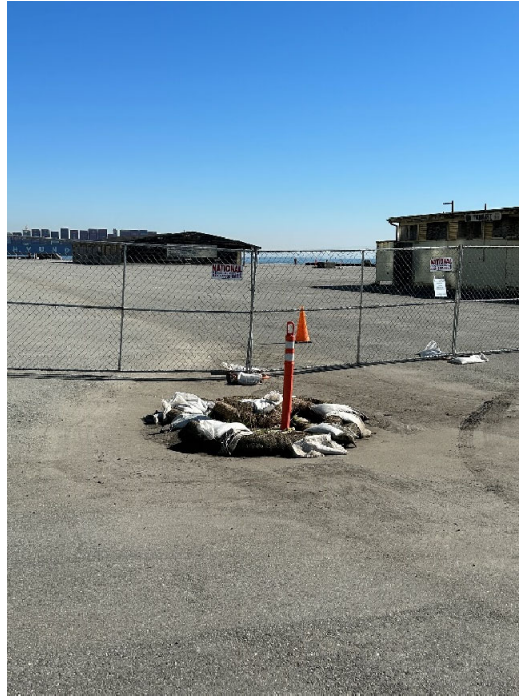
Parcel C Photograph 9: Stormwater best management practices around catch basins during active trenching work. Facing northwest.
