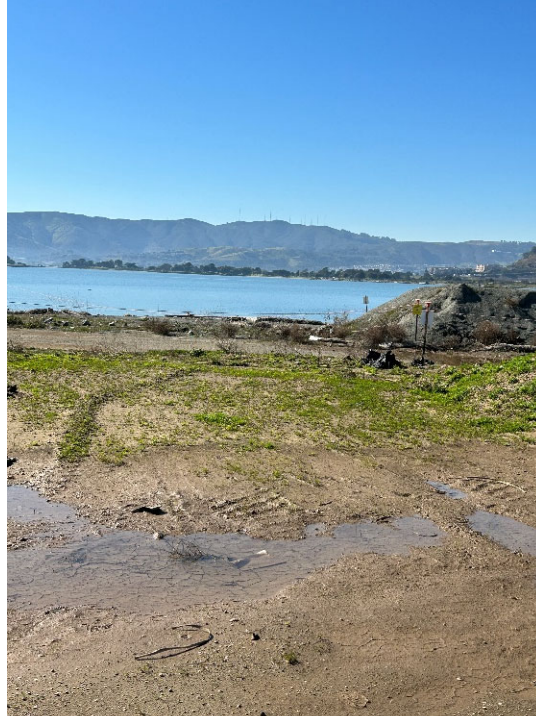
Parcel E Photograph 5: Stockpile with standing water at corner of J and Mahan Street. Facing southwest.
