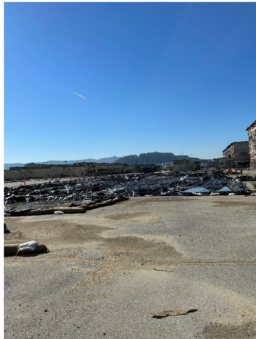
Parcel G Photograph 2: Stormwater best management practice southeast of Building 402. Facing southwest. Photographed by: Marcella Navas/CH2M, 2/9/2023
