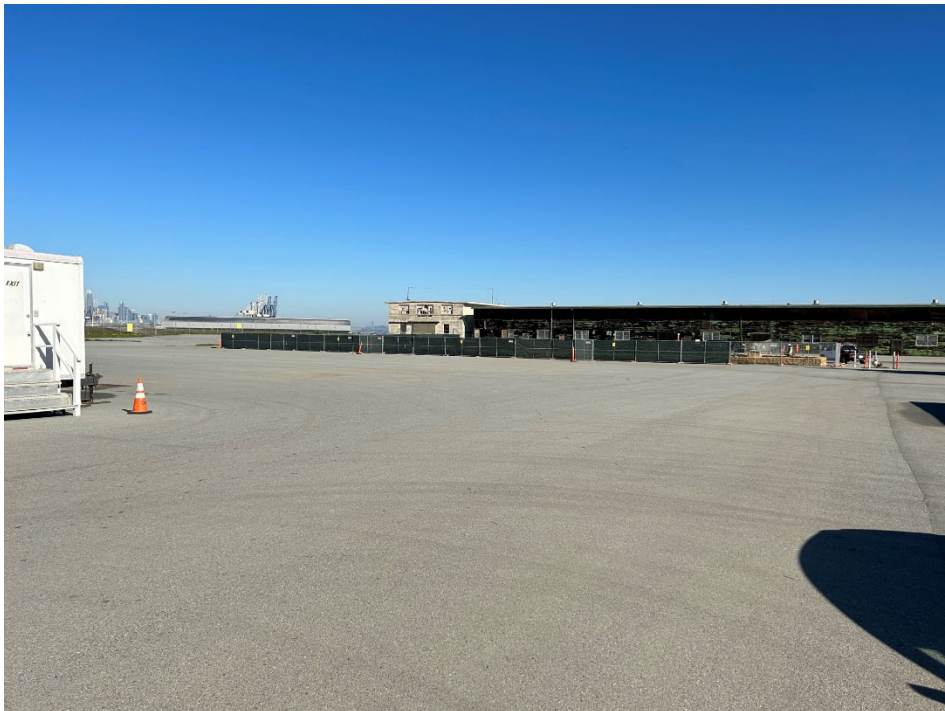
Parcel B-1 Photograph 4: Asphalt pavement cover southeast of Building 121. Facing northwest.
