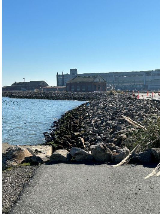
Parcel B-2 Photograph 7: Shoreline revetment southwest of Building 140. Facing southeast.
