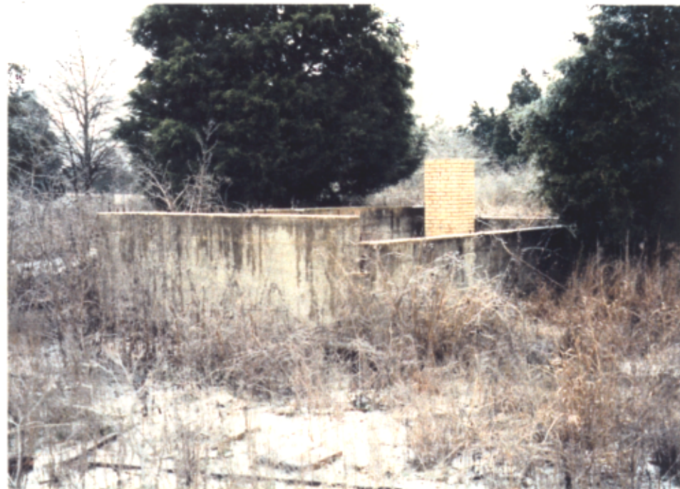
J-6 Area B - old building foundation
