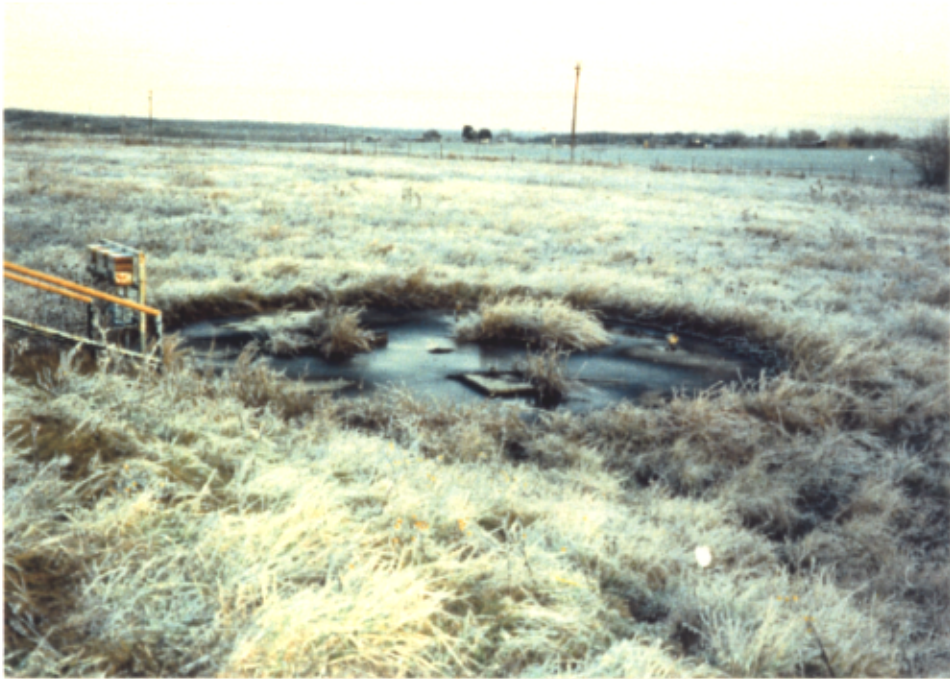
J-17 A type of platform or pad inside potential FUDS on route 2136
