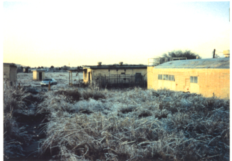
J-16 Abandoned structures at potential FUDS on route 2136
