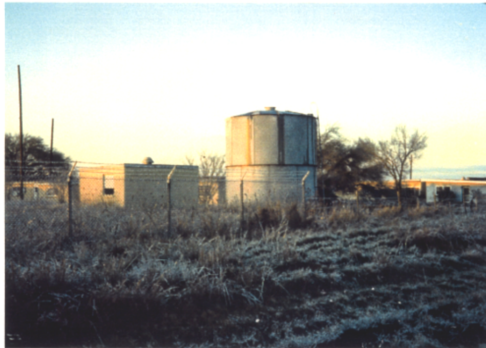
J-19 View of abandoned installation - potential FUDS, from route 2136
