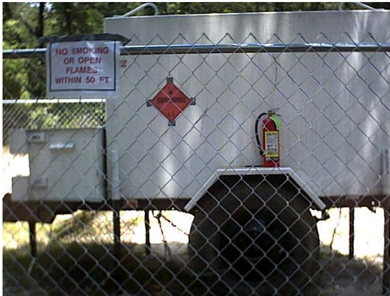
Photograph 3.5 Explosives Storage Magazine
