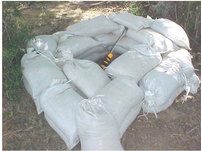
Photograph 3.4 Sandbag Setup for UXO Detonation
