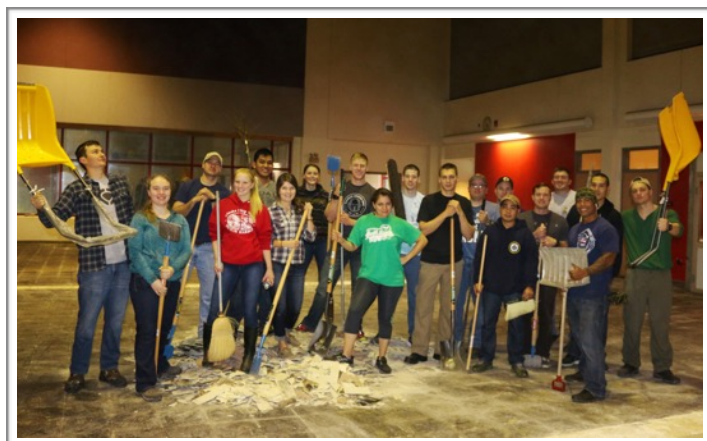
Tile removal crew in the Adak school building.
