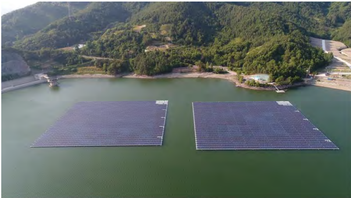
Photo of floating solar cells Geumjeon floating power plant in South Korea.
