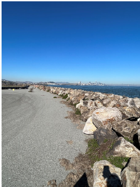
Parcel B-2 Photograph 8: Shoreline revetment north of Building 140. Facing west.
