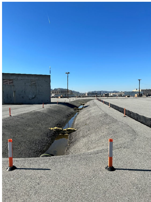
Parcel C Photograph 10: Paved drainage swale outfall south of Building 230. Facing southwest.
