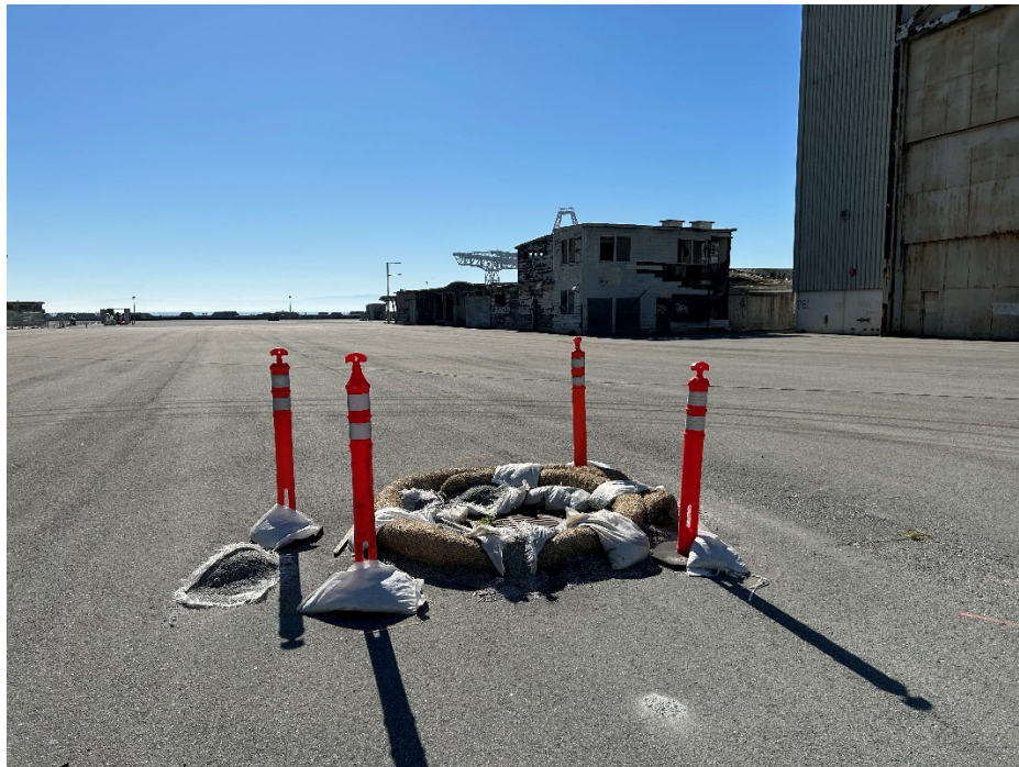
Parcel C Photograph 12: Stormwater best management practice around catch basin west of Building 231. Facing southeast.
