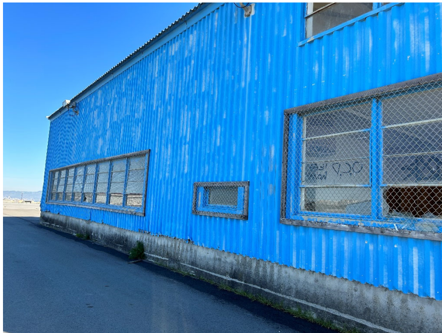
Parcel D-1 Photograph 10: Building 381, vegetation growth in the seam between exterior cover and building foundation. Facing northeast.
