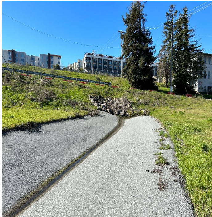
Parcel B-1 Photograph 14: Drainage swale in asphalt pavement cover southwest of Building 120. Facing southwest.
