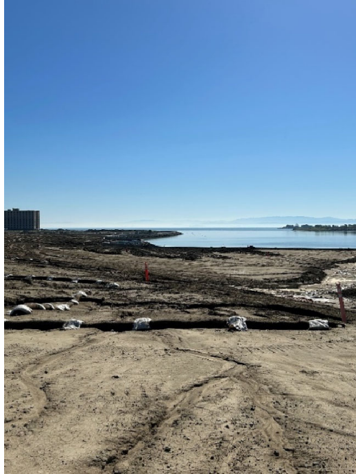
Parcel E-2 Photograph 1: Active construction with stormwater best management practices. Facing southeast.
