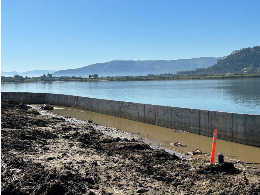
Parcel E-2 Photograph 9: Accumulated water behind seawall in active construction area. Facing southeast.
