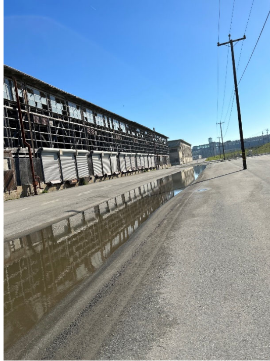
Parcel B-1 Photograph 7: Drainage swale in asphalt pavement cover southwest of Building 123, with accumulation of water. Facing southeast.
