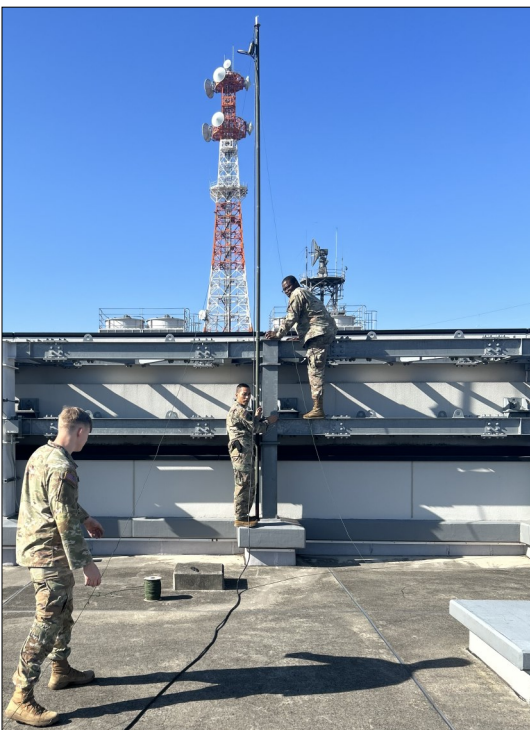
The CPP team installing a Sloping V antenna.
