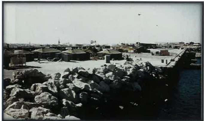
PSU-301 compound on the pier at the Jubail Commercial Port, Al-Jubail, Saudi Arabia ~ Photo: PSU301
