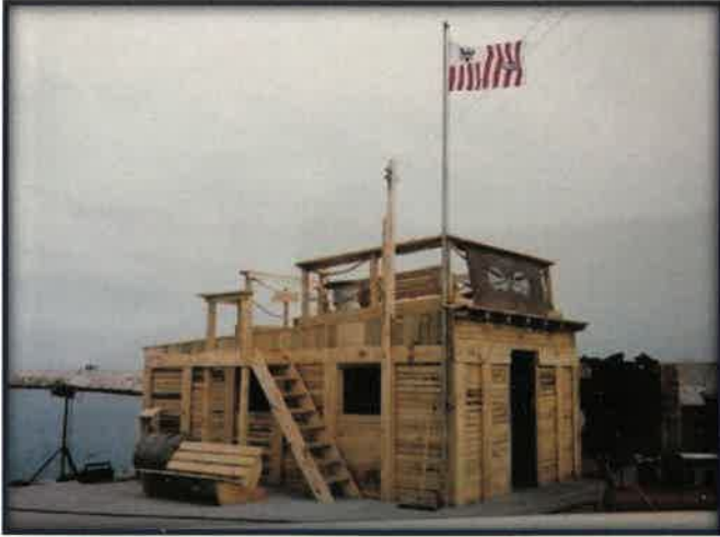
PSU-301 Boat House at Jubail Commercial Port constructed from discarded dunnage ~ Photo: PSU-301
