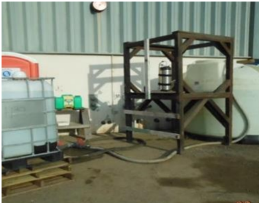
Environmentally-friendly bacteria was used to treat groundwater at IR-10
