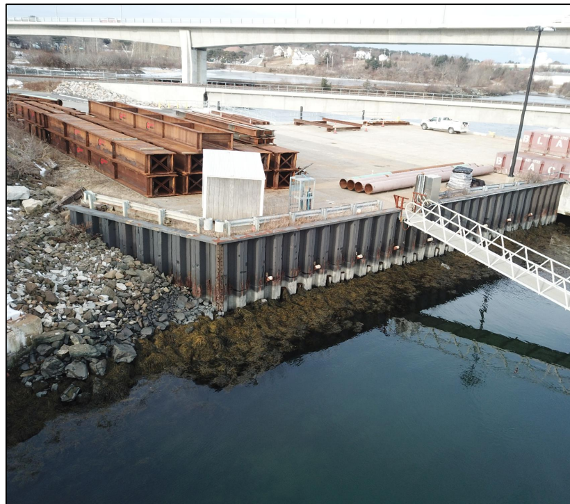
BARGE WHARF BULKHEAD LOOKING WEST (A1)
