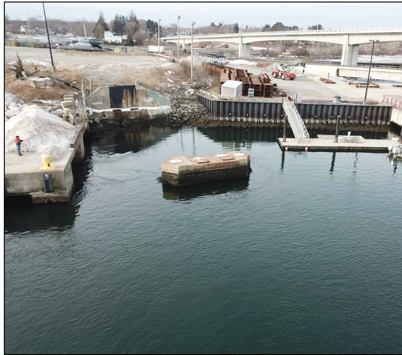
NORTH WHARF EXTENSION LOCATION LOOKING SOUTHWEST (C1)
