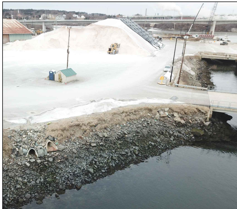
SOUTH WHARF EXTENSION REVETMENT LOOKING WEST
