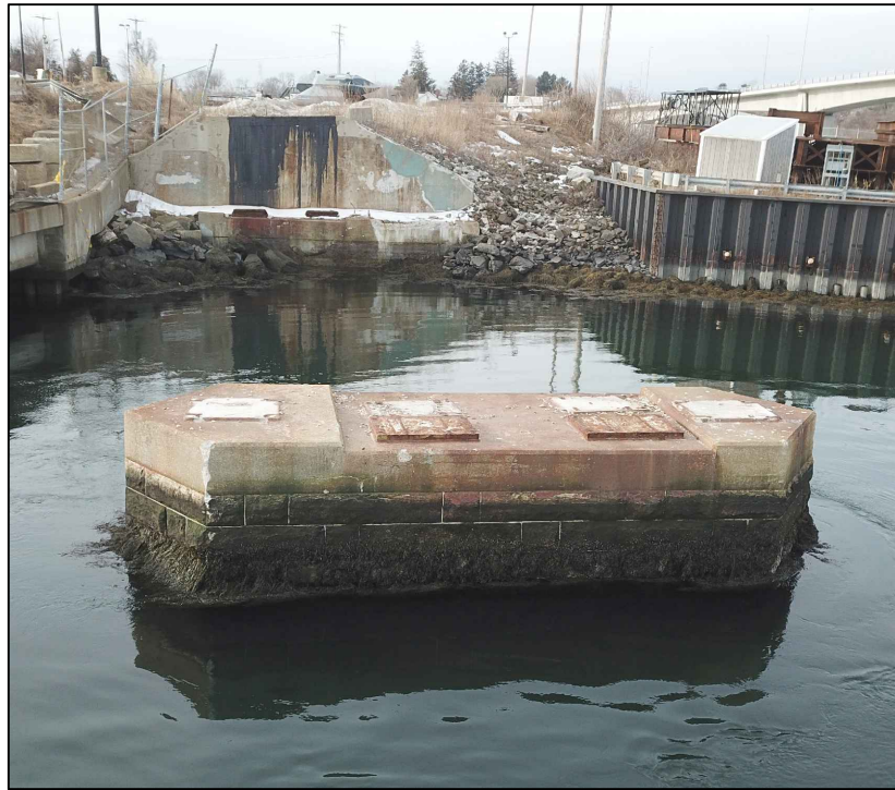
BRIDGE PIER 14 LOOKING SOUTHWEST (C3)
