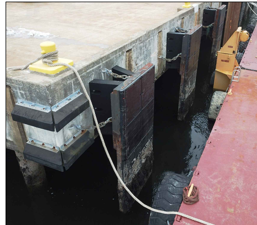
BARGE WHARF - FENDER SYSTEM LOOKING SOUTH
