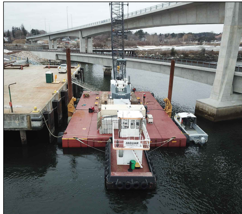
FLOATING DOCK - NEW LOCATION LOOKING SOUTHWEST (A4)
