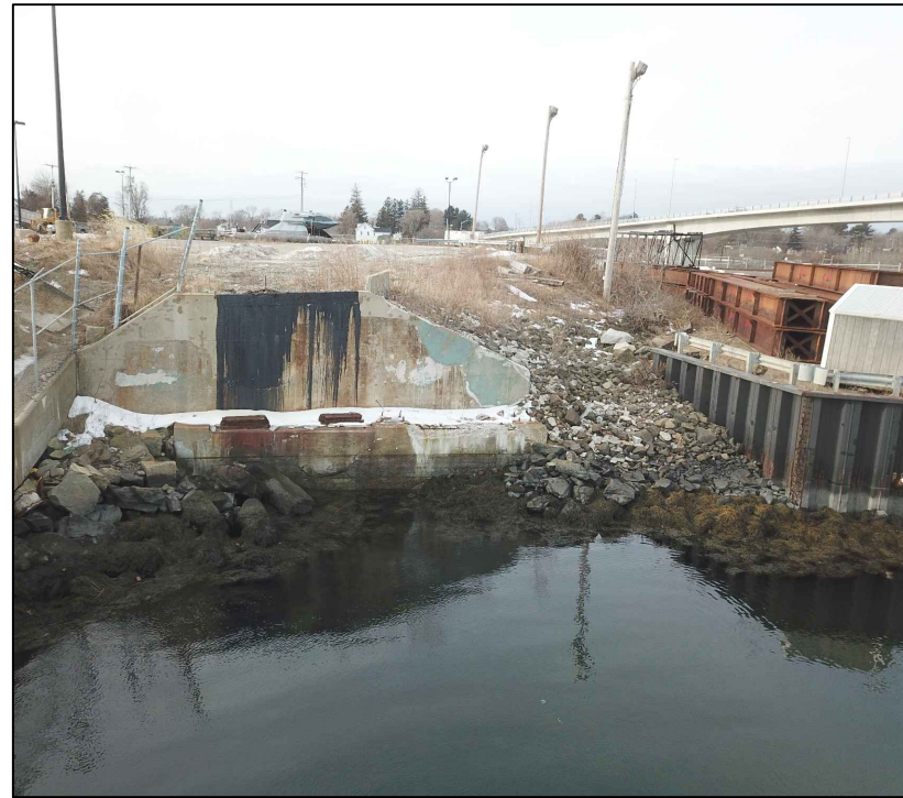
BRIDGE ABUTMENT 13 LOOKING SOUTHWEST (C4)
