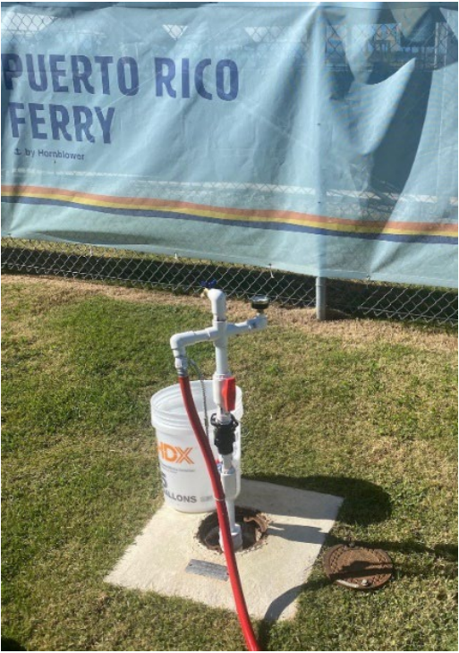
Injection Wellhead
