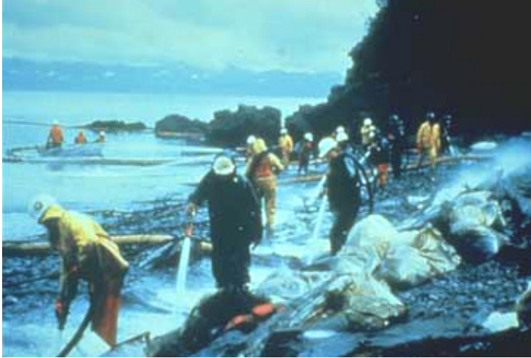
When crews cleaned a beach with high-pressure, hot-water washing, booms were used, as shown here, to prevent oil refloated by the cleaning operations from escaping back into Prince William Sound.
