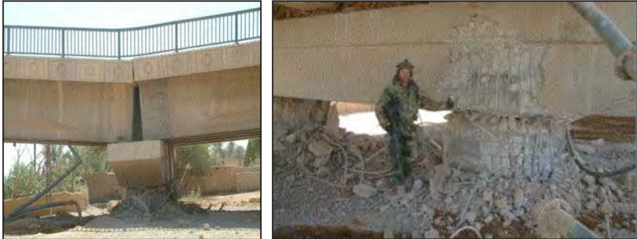
Figure 6: Bridge at Al Kifl 6
