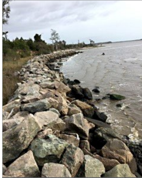
Figure 4. Rock Installed Along the Cape Fear River Source: The DoD OIG.
