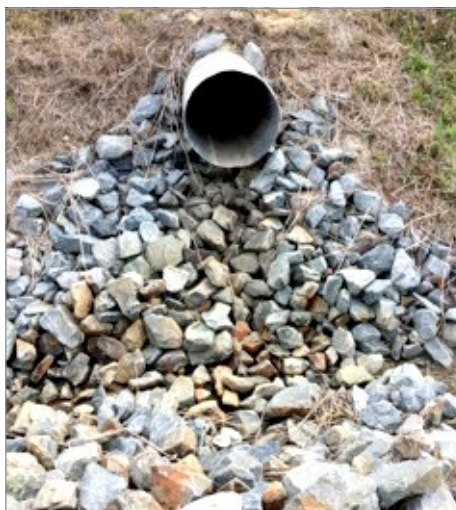
Figure 2. Updated Culvert with Installed Rock at MOTSU Source: The DoD OIG.
