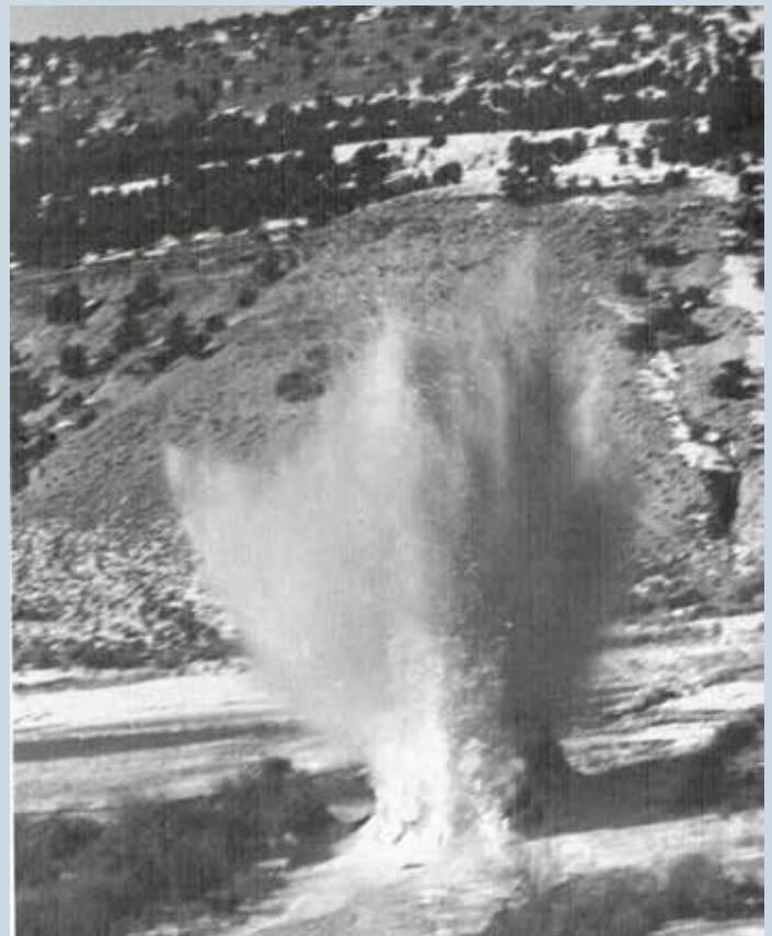
Utah National Guard Soldiers from Company A, 1457th Engineer Battalion, use more than 850 pounds of explosives to clear an ice jam on the Strawberry River, enabling the river to flow once again.
