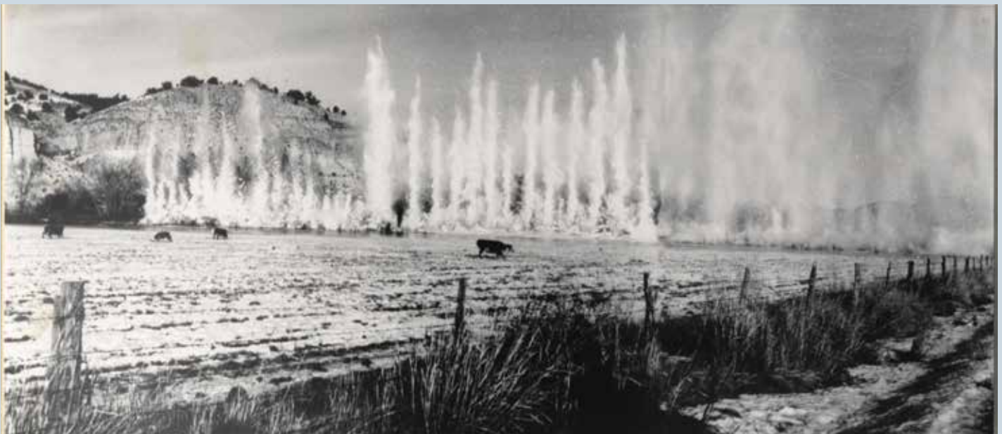
Utah National Guard Soldiers from Company A, 1457th Engineer Battalion, use more than 850 pounds of explosives to clear an ice jam on the Strawberry River, enabling the river to flow once again.
