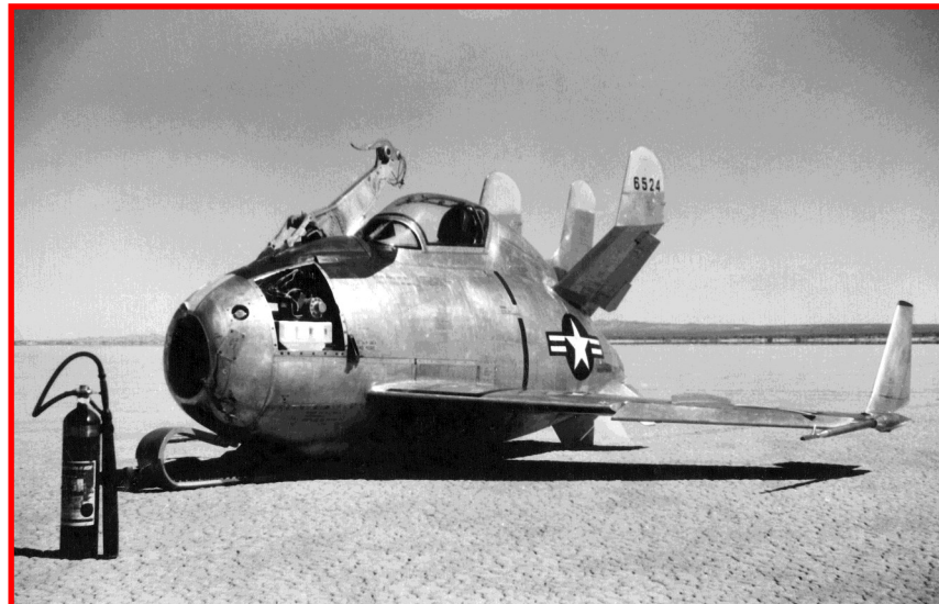
XF-85, 46-524 sits on the lakebed after it's sixth, and final, flight on 18 March, 1949. The 19 minute flight tested the redesigned nose hook and added winglets mounted on the outboard wings.
