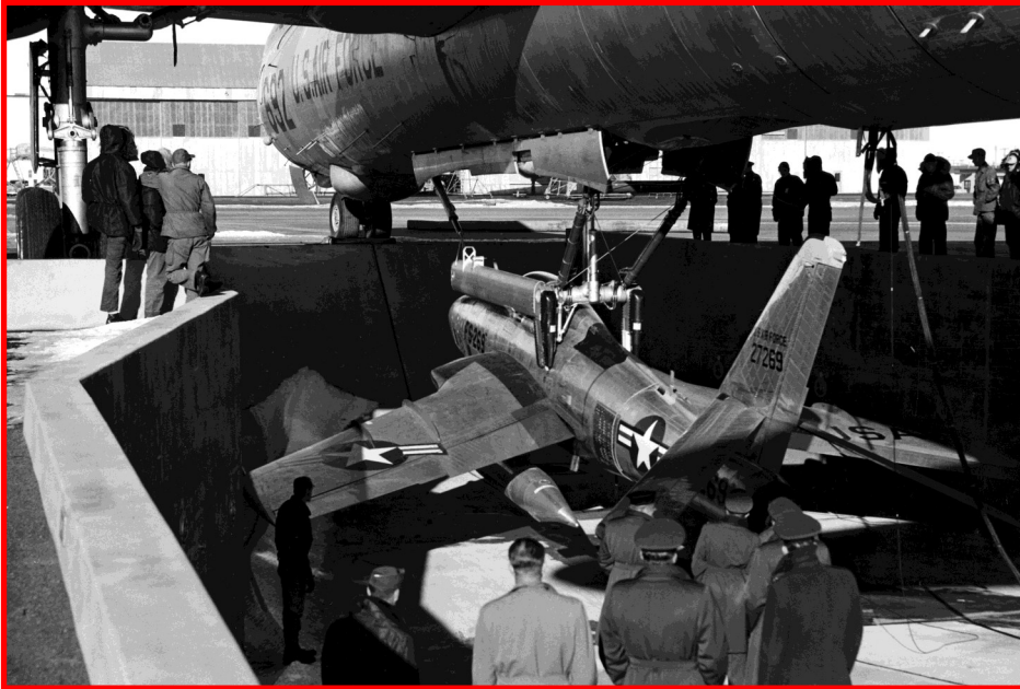
Operational RF-84K parasites were loaded into the GRB-36D via a special concrete pit constructed at Fairchild AFB, WA.
