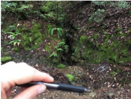
Photo 1. Culvert inlet (March 2021).
