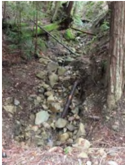
Photo 1. Culvert inlet area (March 2021).
