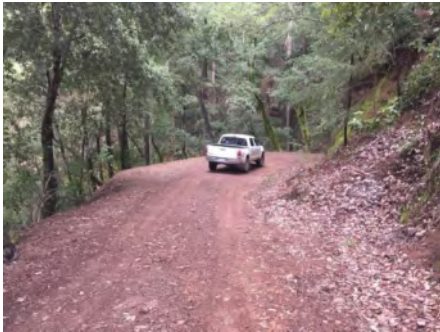
Photo 1. Culvert inlet buried beneath slide at right (March 2021) .
