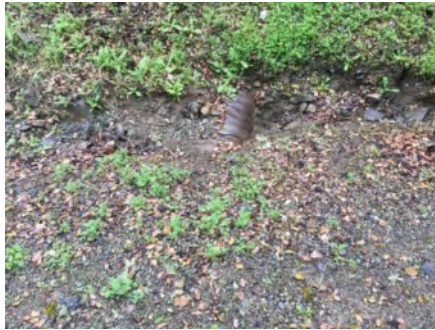
Photo 2. Culvert outlet ( March 2021 ).
