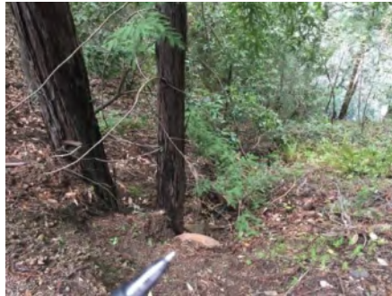
Photo 2. Culvert outlet area ( March 2021 ).
