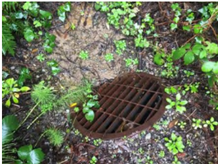
Photo 1. Culvert inlet area (March 2021).
