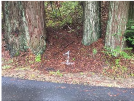
Photo 1. Culvert inlet area, as indicated by spray paint mark ( March 2021 ).
