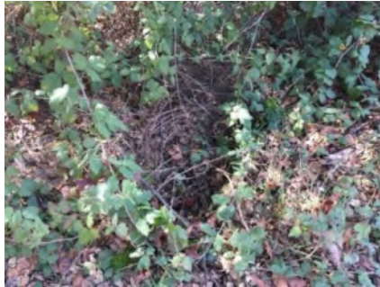
Photo 2. Culvert outlet area (Jan 2019).
