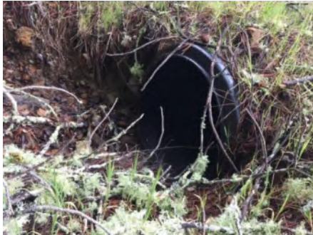
Photo 1. Culvert inlet ( March 2021 ).
