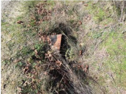
Photo 1. Culvert inlet area (Jan 2019).
