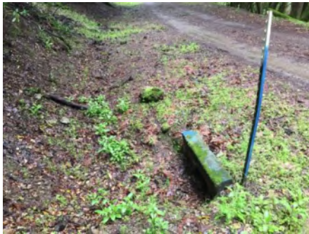
Photo 1. Culvert inlet area ( March 2021 ).
