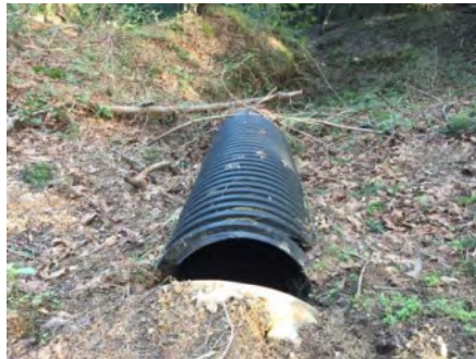
Photo 2. Culvert outlet (Jan 2019).
