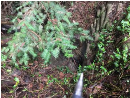
Photo 1. Culvert inlet area (March 2021).
