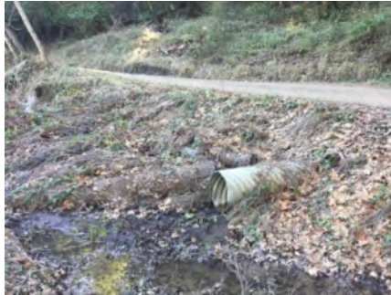
Photo 2. Culvert outlet (Jan 2019).
