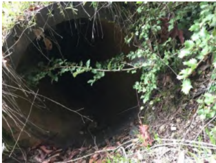
Photo 1. Culvert inlet ( March 2021 ).
