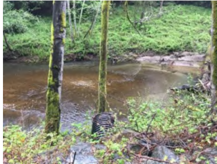
Photo 2. Culvert outlet ( March 2021 ).
