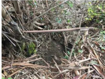
Photo 2. Culvert outlet ( March 2021 ).
