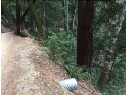
Photo 2. Culvert outlet (Jan 2019).
