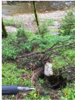
Photo 2. Culvert outlet (March 2021).
