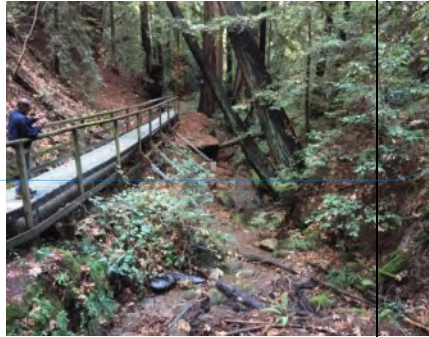
Photo 50. View downstream of Howell Intake Facility (Dec. 2018).
