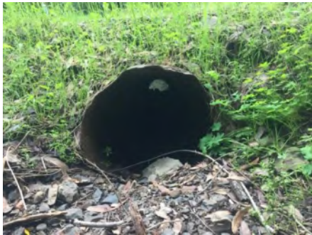
Photo 1. Culvert inlet area ( March 2021 ).
