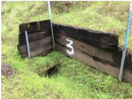
Photo 1. Culvert inlet area (March 2021).
