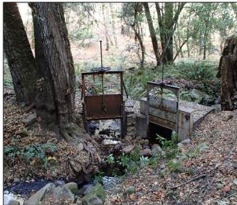
Photo 14. Creek “splitter” gates northwest of Lake Ranch Reservoir (Dec. 2013).
