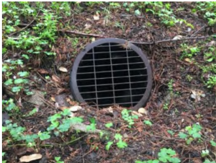
Photo 1. Culvert inlet area (March 2021).
