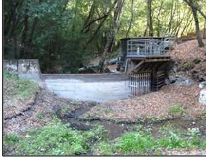
Photo 24. Hooker Intake Facility (May 2013).
