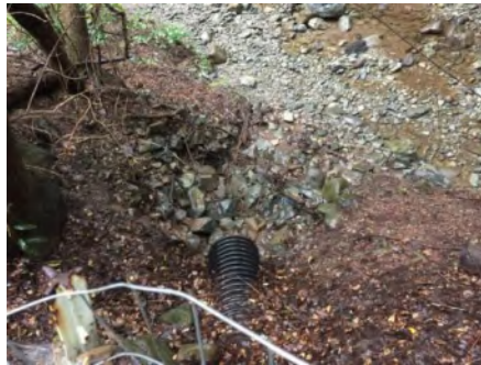
Photo 2. Culvert outlet (March 2021).
