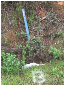
Photo 1. Culvert inlet ( March 2021 ).
