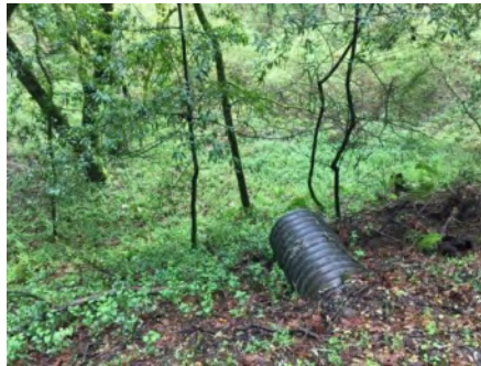
Photo 2. Culvert outlet ( March 2021 ).
