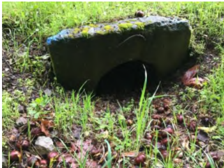
Photo 1. Culvert inlet area (March 2021).
