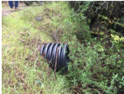
Photo 2. Culvert outlet ( March 2021 ).
