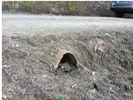
Photo 2. Culvert outlet (Jan 2019).
