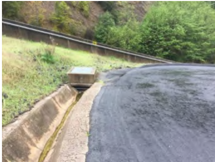
Photo 1. Culvert inlet (March 2021).
