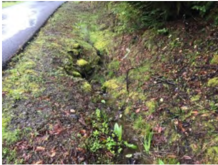
Photo 1. Culvert inlet (March 2021).
