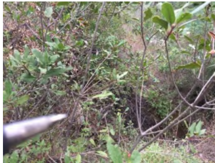
Photo 2. Culvert outlet ( March 2021 ).
