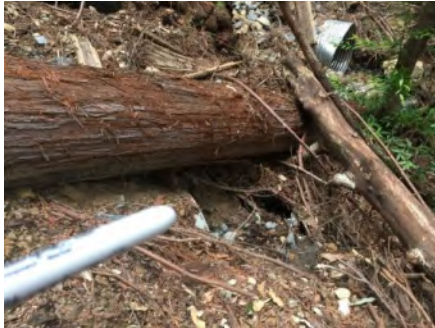
Photo 2. Culvert outlet (Jan 2019).
