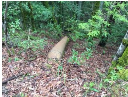
Photo 2. Culvert outlet ( March 2021 ).
