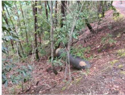
Photo 2. Culvert outlet (March 2021).
