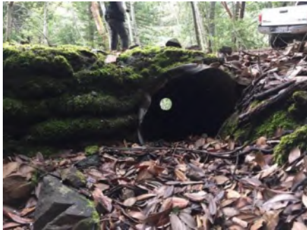
Photo 1. Culvert inlet (March 2021).
