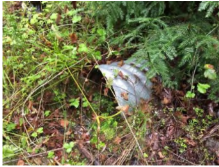
Photo 2. Culvert outlet ( March 2021 ).
