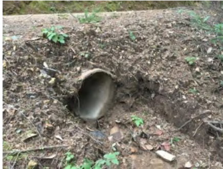
Photo 2. Culvert outlet (Jan 2019).
