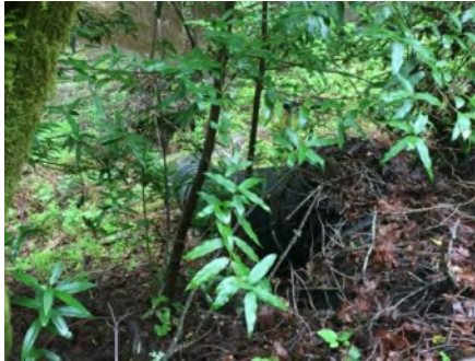
Photo 2. Culvert outlet ( March 2021 ).
