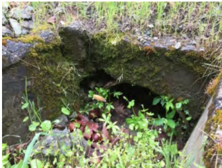
Photo 1. Culvert inlet area ( March 2021 ).
