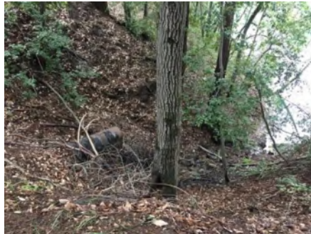
Photo 2. Culvert outlet ( March 2021 ).
