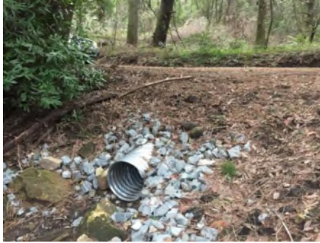
Photo 2. Culvert outlet (Jan 2019).
