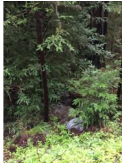
Photo 2. Culvert outlet (March 2021).
