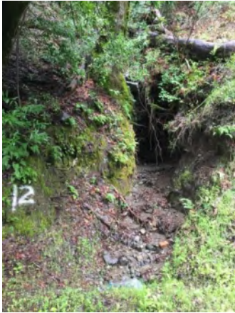
Photo 1. Culvert inlet area (March 2021).
