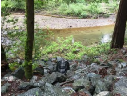
Photo 2. Culvert outlet (March 2021).
