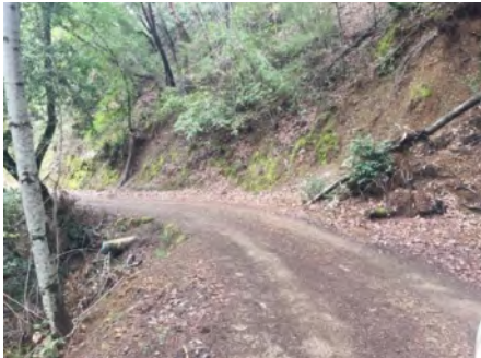
Photo 1. Culvert inlet buried beneath slide ( March 2021 ).
