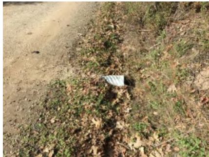
Photo 1. Culvert inlet area (Jan 2019).
