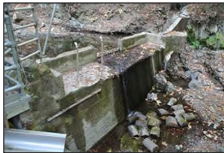
Photo 39. Notched weir of the Beardsley Creek Intake Facility (Oct. 2013).
