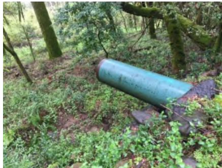
Photo 2. Culvert outlet (March 2021).
