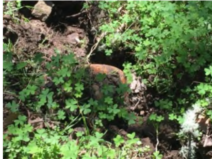
Photo 2. Culvert outlet (Mar. 2014).
