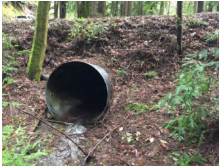
Photo 1. Culvert inlet ( March 2021 ).
