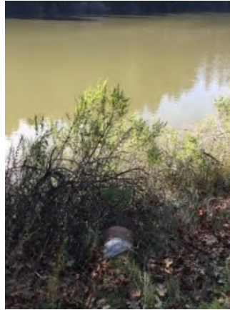
Photo 2. Culvert outlet area (Jan 2019).
