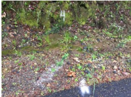
Photo 1. Culvert inlet ( March 2021 ).
