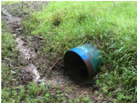
Photo 1. Culvert inlet area (March 2021).
