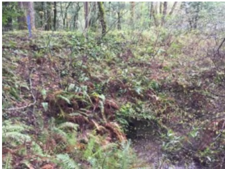
Photo 1. Culvert inlet area (March 2021).
