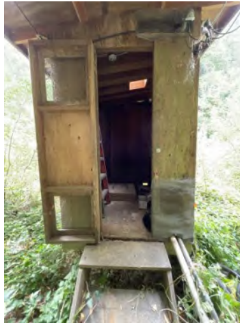
Photo 52. Aldercroft Heights Extraction Well pump house (Aug. 2021)
