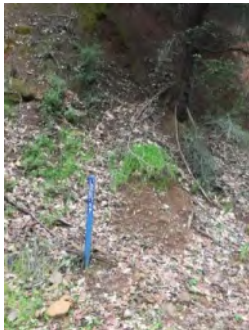
Photo 1. Culvert inlet ( March 2021 ).
