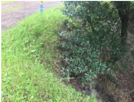
Photo 2. Culvert outlet ( March 2021 ).
