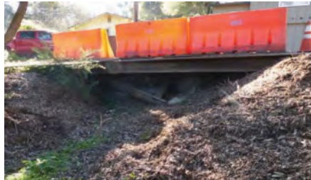
Photo 2. Culvert outlet (April 2019).
