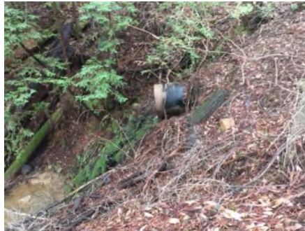
Photo 2. Culvert outlet ( March 2021 ).
