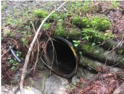
Photo 2. Culvert outlet (March 2021).
