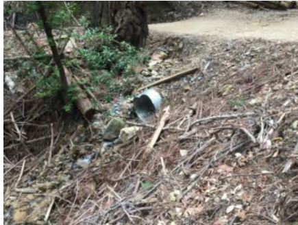
Photo 2. Culvert outlet (Jan 2019).
