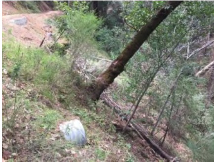
Photo 2. Culvert outlet (Jan 2019).
