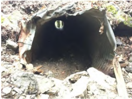
Photo 1. Culvert inlet (March 2021).
