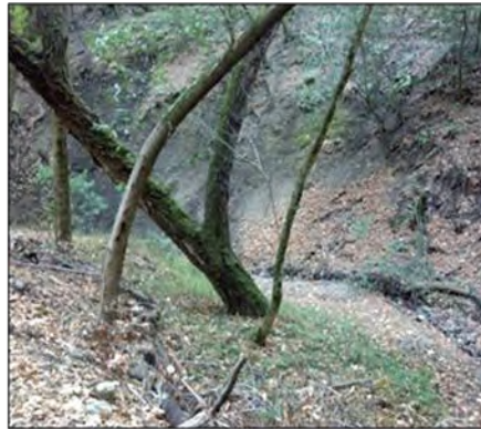
Photo 34. Looking upstream from Hendry Intake Facility (Dec. 2013).
