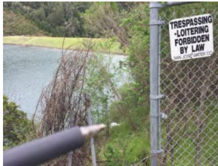
Photo 2. Culvert outlet ( March 2021 ).
