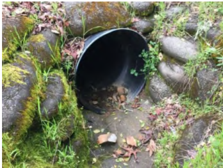
Photo 1. Culvert inlet ( March 2021 ).
