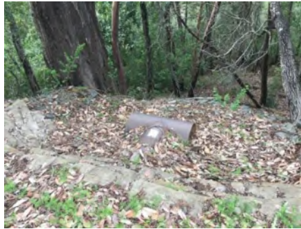
Photo 2. Culvert outlet ( March 2021 ).
