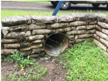
Photo 1. Culvert inlet ( March 2021 ).
