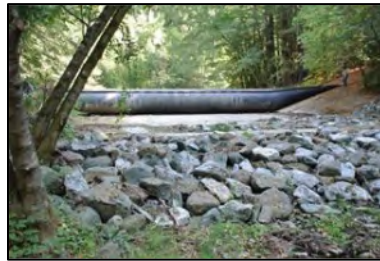
Photo 21. Inflatable dam at Ostwald Intake (Dec. 2013).
