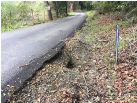
Photo 1. Culvert inlet ( March 2021 ).
