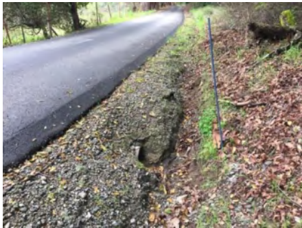
Photo 1. Culvert inlet (March 2021).
