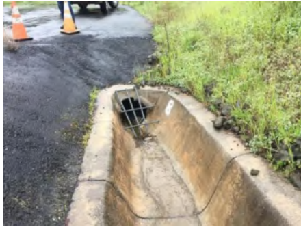
Photo 1. Culvert inlet (March 2021).
