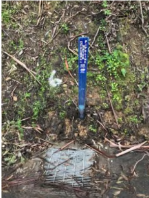
Photo 1. Culvert inlet (March 2021).
