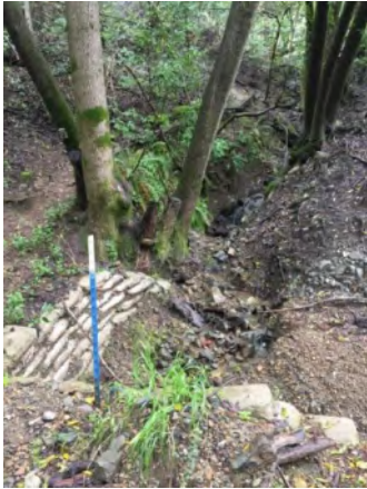
Photo 1. Culvert inlet area (March 2021).
