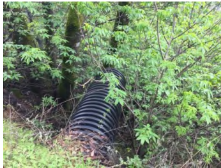
Photo 2. Culvert outlet ( March 2021 ).
