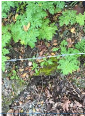
Photo 2. Culvert outlet ( March 2021 ).
