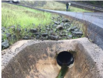
Photo 2. Culvert outlet (March 2021).
