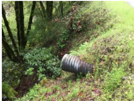
Photo 2. Culvert outlet (March 2021).
