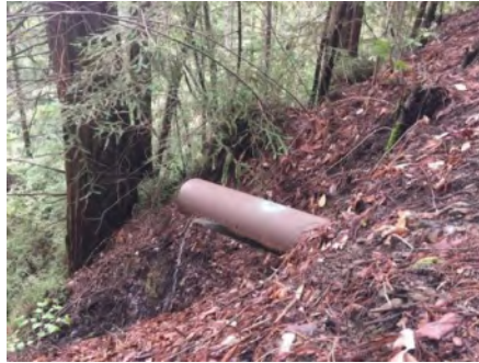
Photo 2. Culvert outlet ( March 2021 ).
