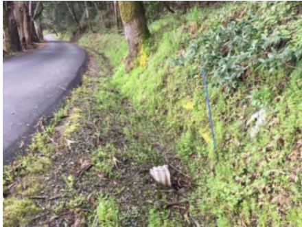
Photo 1. Culvert inlet (March 2021).
