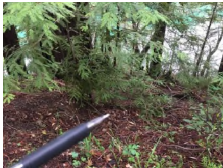
Photo 2. Culvert outlet ( March 2021 ).
