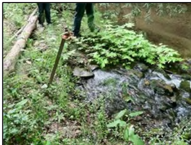
Photo 18. Discharge pipe maintaining 2 cfs downstream of Ostwald Intake (Oct. 2013).
