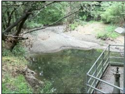
Photo 25. Sediment deposited upstream of Hooker Intake Facility (May 2013).
