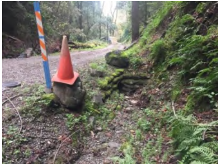
Photo 1. Culvert inlet area (March 2021).
