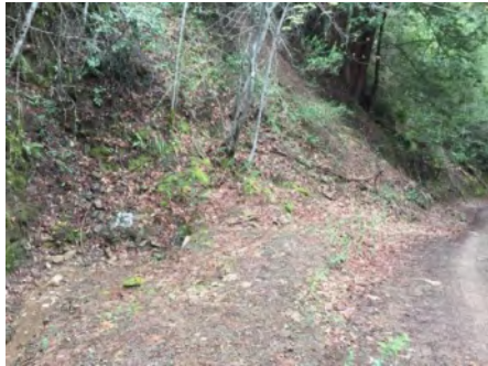
Photo 1. Culvert inlet area at left (March 2021) .
