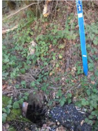
Photo 2. Culvert outlet area (Jan 2019).
