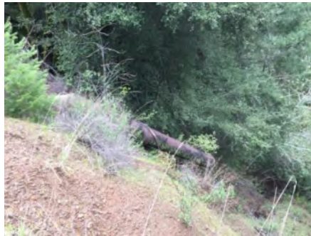
Photo 2. Culvert outlet ( March 2021 ).
