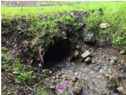
Photo 1. Culvert inlet area (March 2021).
