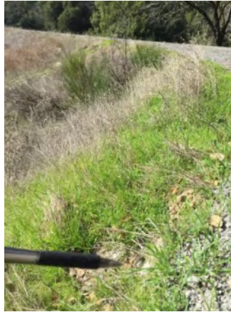
Photo 2. Culvert outlet area (Jan 2019).
