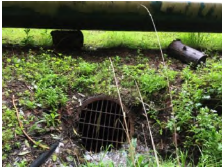
Photo 1. Culvert inlet area ( March 2021 ).
