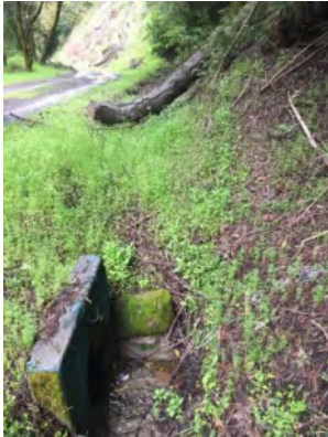
Photo 1. Culvert inlet area ( March 2021 ).
