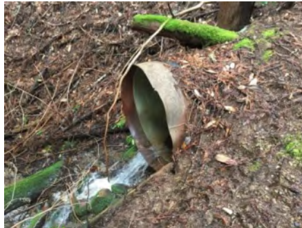
Photo 2. Culvert outlet (March 2021).
