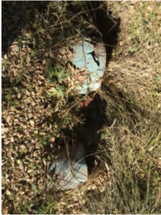
Photo 1. Culvert M27 and M28 inlets (Jan 2019).
