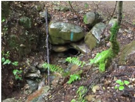
Photo 1. Culvert inlet area (March 2021).
