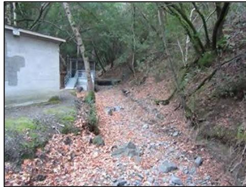
Photo 43. Trout Creek Intake Facility weir and intake in distance, pump house to left (Oct. 2013).
