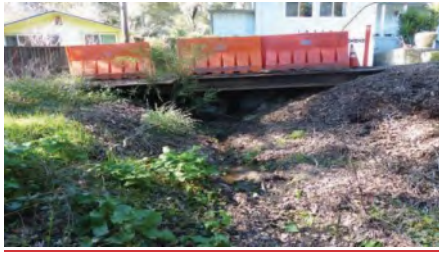
Photo 1. Culvert outlet area (April 2019).
