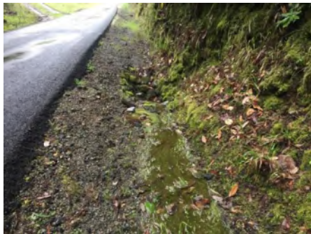
Photo 1. Culvert inlet ( March 2021 ).
