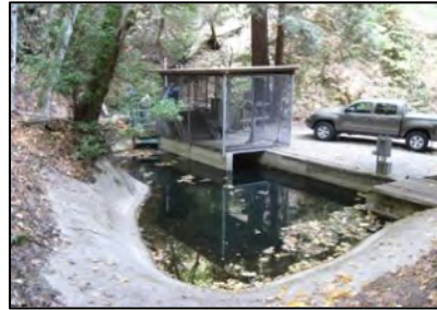
Photo 40. Storage pool, intake gate, and leaf/debris screening device (Oct. 2013).
