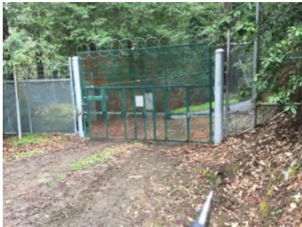
Photo 1. Culvert inlet ( March 2021 ).
