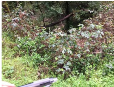
Photo 2. Culvert outlet area (March 2021).
