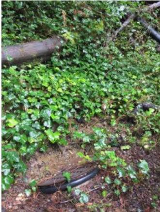
Photo 1. Culvert inlet area (March 2021).
