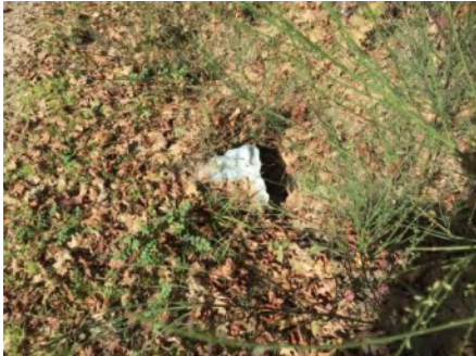
Photo 1. Culvert inlet area (Jan 2019).
