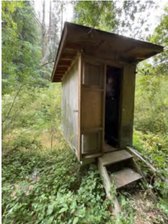
Photo 51. Aldercroft Heights Extraction Well pump house (Aug. 2021)
