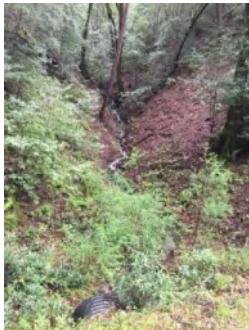
Photo 1. Culvert inlet ( March 2021 ).
