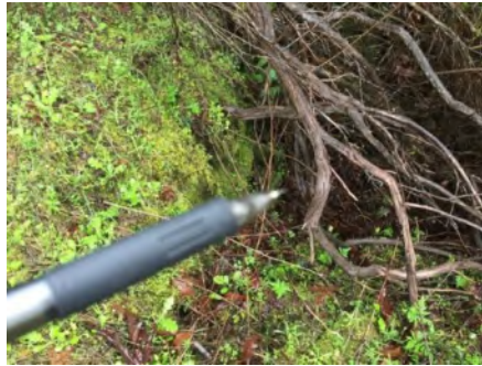
Photo 2. Culvert outlet (March 2021).
