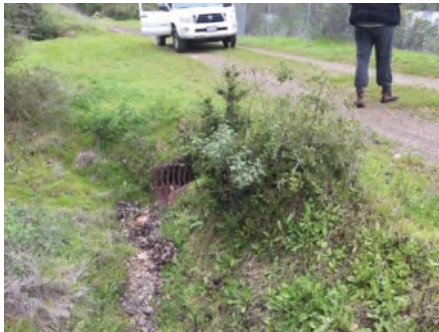
Photo 1. Culvert inlet ( March 2021 ).
