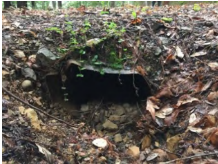
Photo 1. Culvert inlet (March 2021).
