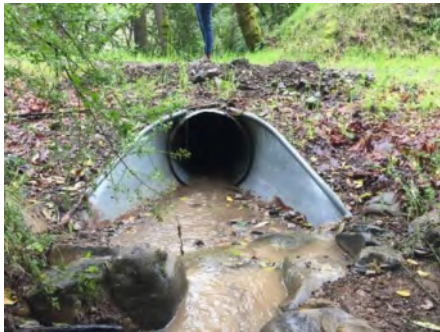
Photo 1. Culvert inlet area (March 2021).
