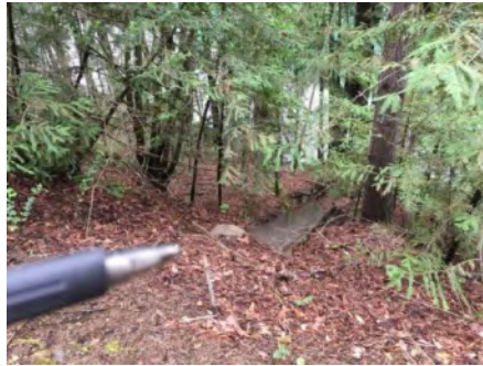
Photo 2. Culvert outlet (March 2021) .
