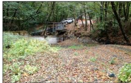
Photo 30. Upstream side of Hooker Intake and dam (Nov. 2013).
