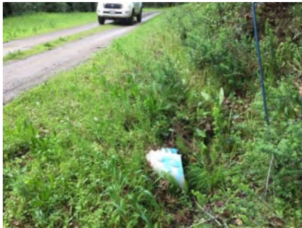
Photo 1. Culvert inlet (March 2021).
