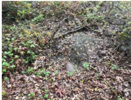
Photo 2. Culvert outlet (March 2021).
