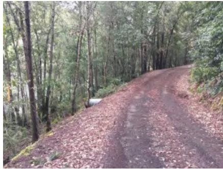
Photo 2. Culvert outlet area at left (March 2021).
