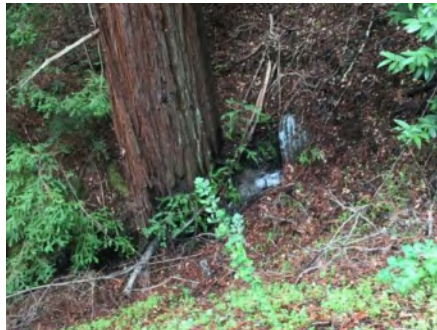
Photo 2. Culvert outlet area. ( March 2021 ).
