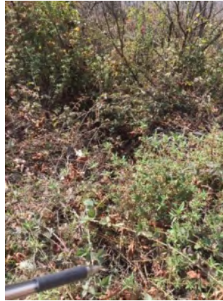
Photo 2. Culvert outlet area (Jan 2019).
