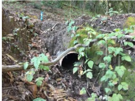
Photo 2. Culvert outlet (Jan 2019).
