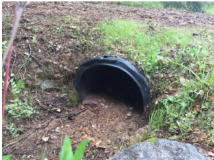
Photo 1. Culvert inlet (March 2021).
