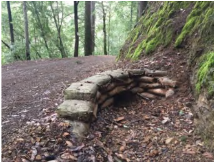
Photo 1. Culvert inlet (March 2021).
