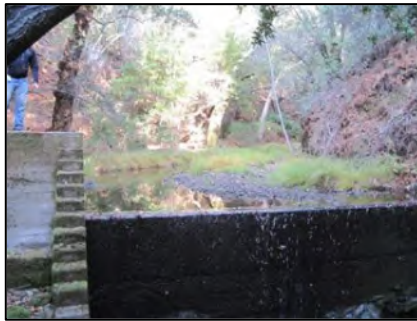
Photo 36. Concrete weir without flashboards in place at Upper Cavaneer Intake (Dec. 2013).
