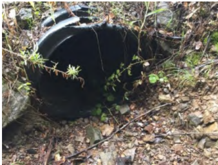
Photo 1. Culvert inlet ( March 2021 ).
