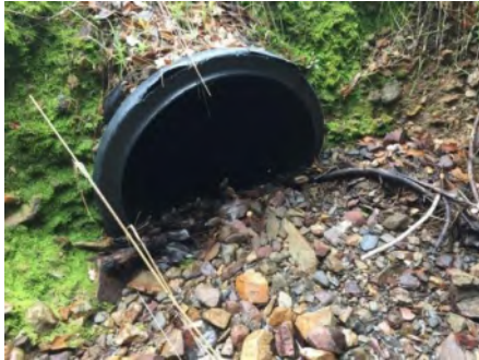
Photo 1. Culvert inlet ( March 2021 ).
