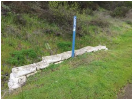
Photo 1. Culvert inlet ( March 2021 ).
