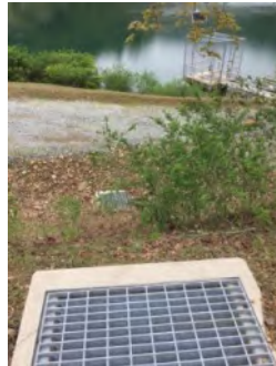
Photo 2. Culvert outlet ( March 2021 ).
