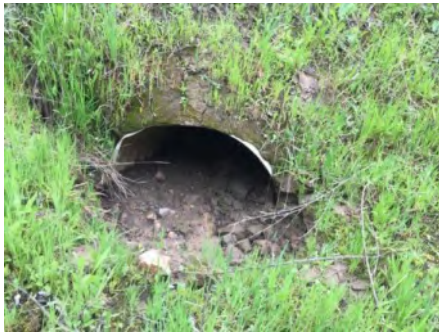
Photo 1. Culvert inlet ( March 2021 ).
