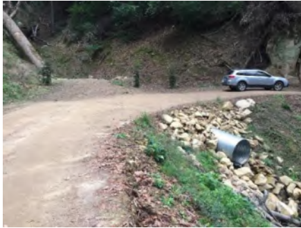
Photo 2. Culvert outlet (Jan 2019).
