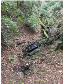
Photo 1. Culvert inlet area ( March 2021 ).
