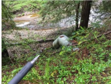
Photo 2. Culvert outlet ( March 2021 ).
