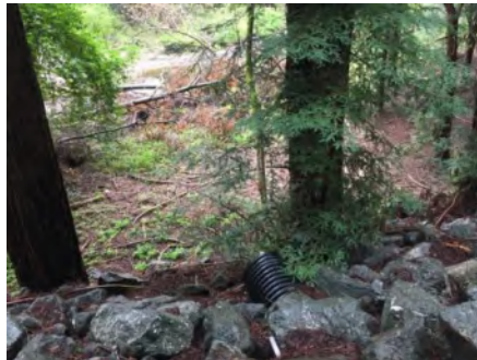
Photo 2. Culvert outlet (March 2021).
