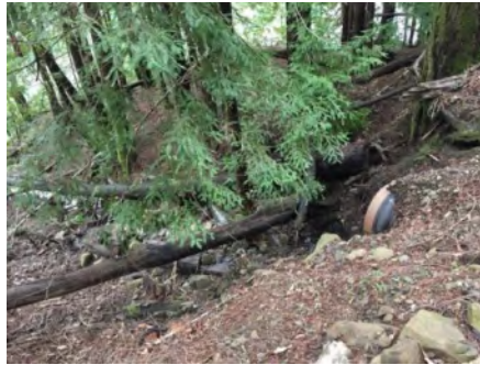
Photo 2. Culvert outlet (March 2021).
