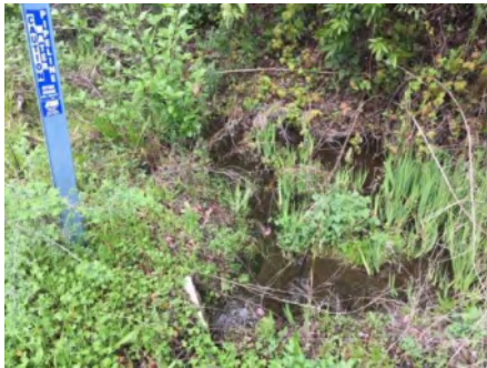
Photo 1. Culvert inlet is below blue marker ( March 2021 ).
