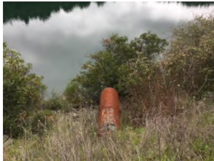
Photo 2. Culvert outlet ( March 2021 ).
