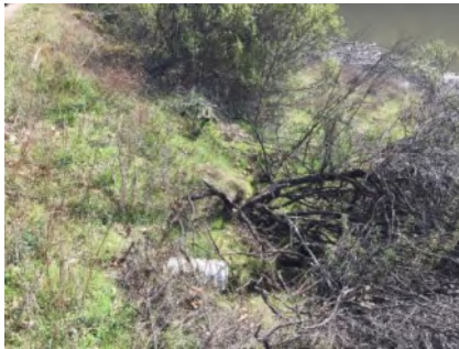
Photo 2. Culvert outlet area (Jan 2019).
