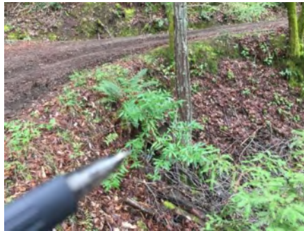
Photo 2. Culvert outlet location indicated by pencil ( March 2021 ).
