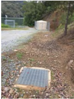
Photo 1. Culvert inlet (March 2021).
