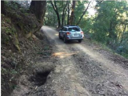
Photo 1. Culvert inlet (Jan 2019).
