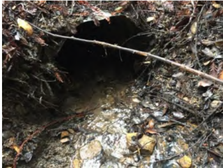
Photo 1. Culvert inlet ( March 2021 ).
