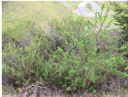
Photo 2. Culvert outlet area ( March 2021 ).
