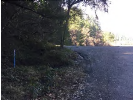
Photo 1. Culvert inlet (Jan 2019).
