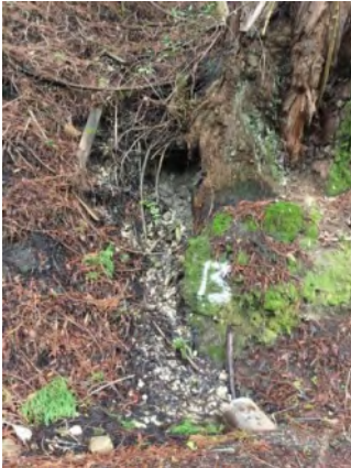
Photo 1. Culvert inlet area (March 2021).
