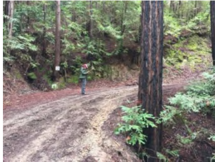
Photo 2. Culvert outlet area is on the slope at right ( March 2021 ).
