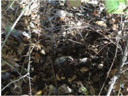
Photo 1. Culvert inlet area (Jan 2019).
