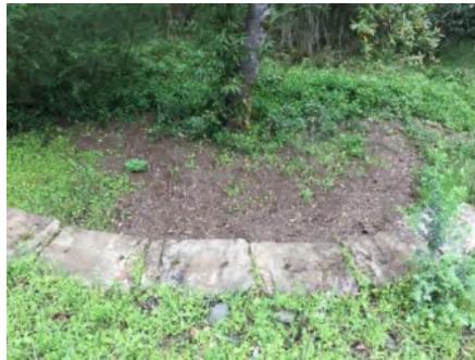
Photo 2. Culvert outlet area. ( March 2021 ).
