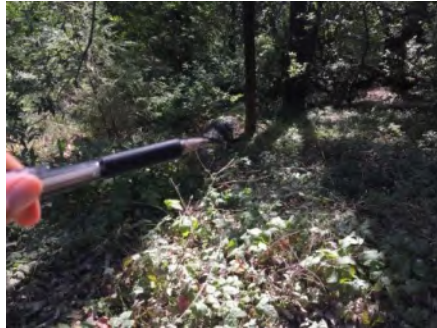
Photo 2. Culvert outlet (Jan 2019).
