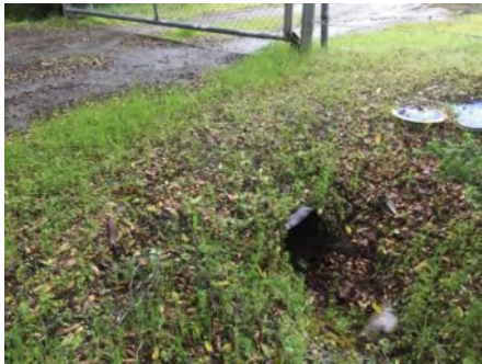
Photo 1. Culvert inlet area ( March 2021 ).
