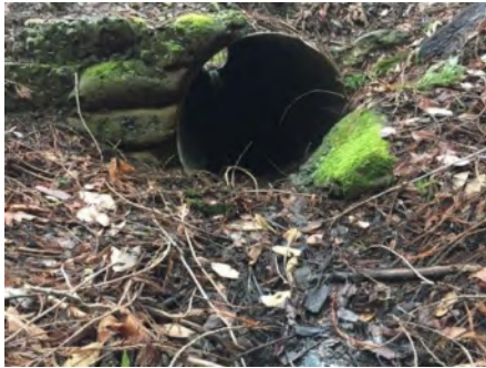
Photo 1. Culvert inlet (March 2021).
