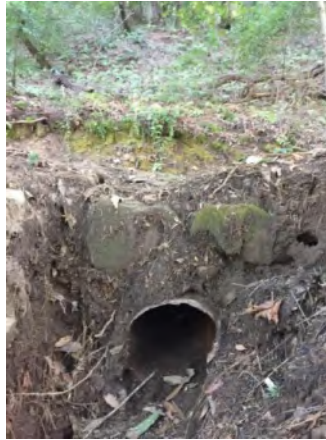
Photo 2. Culvert outlet (Jan 2019).
