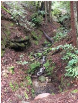
Photo 1. Culvert inlet area (March 2021).
