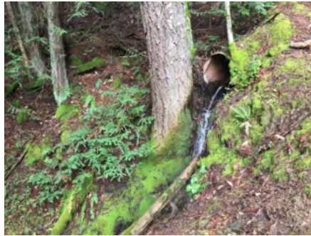
Photo 2. Culvert outlet (March 2021).
