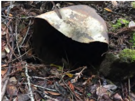
Photo 1. Culvert inlet ( March 2021 ).
