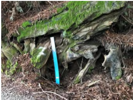
Photo 1. Culvert inlet (March 2021).
