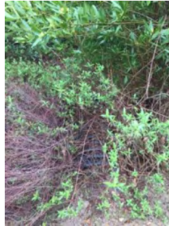
Photo 2. Culvert outlet ( March 2021 ).
