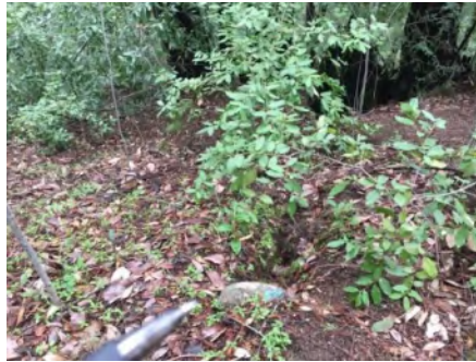
Photo 2. Culvert outlet (March 2021).
