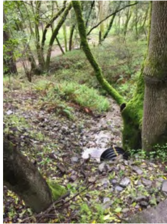
Photo 2. Culvert outlet (March 2021).
