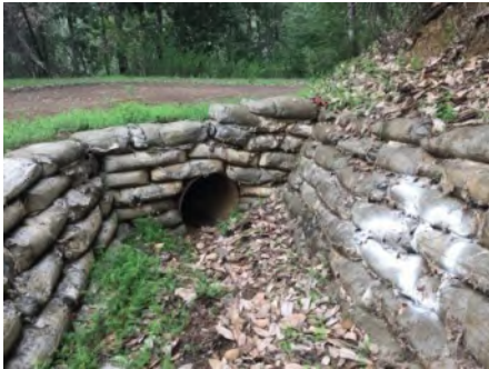
Photo 1. Culvert inlet ( March 2021 ).
