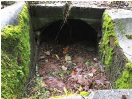
Photo 1. Culvert inlet area (March 2021).
