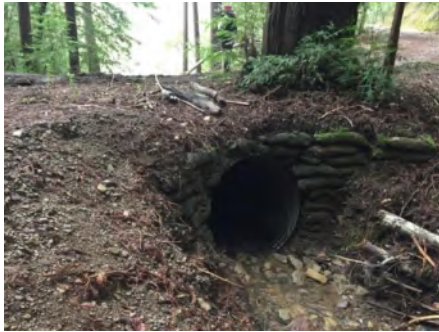
Photo 1. Culvert inlet (March 2021).
