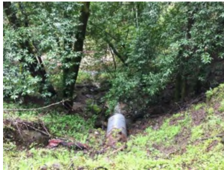
Photo 2. Culvert outlet (March 2021).
