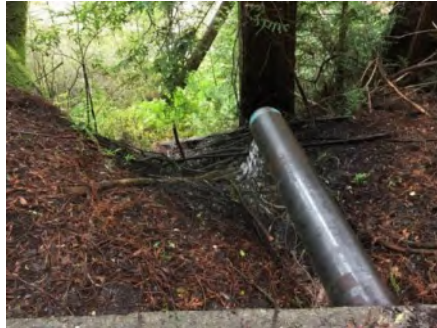
Photo 2. Culvert outlet (March 2021).
