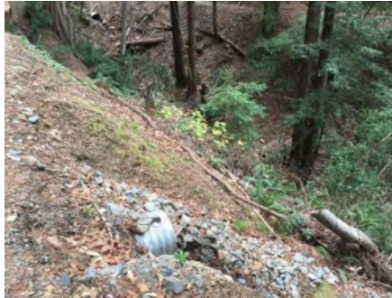
Photo 2. Culvert outlet (Jan 2019).
