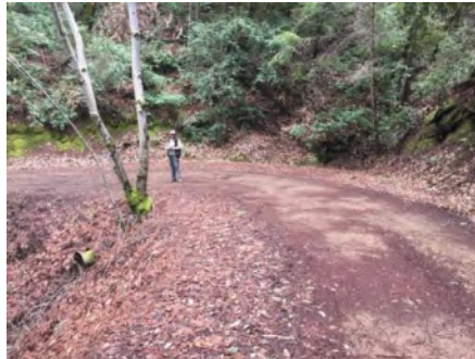
Photo 2. Culvert outlet area at left (March 2021).
