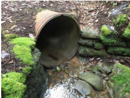
Photo 1. Culvert inlet area ( March 2021 ).
