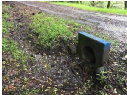
Photo 1. Culvert inlet area (March 2021).
