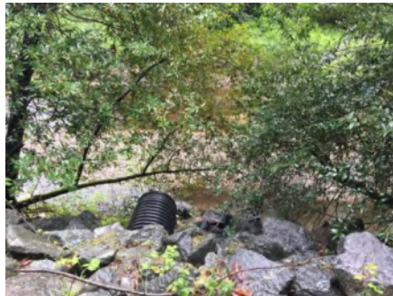
Photo 2. Culvert outlet (March 2021).
