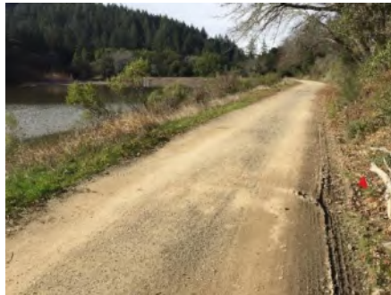
Photo 2. Culvert outlet area (Jan 2019).
