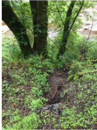
Photo 2. Culvert outlet (March 2021).
