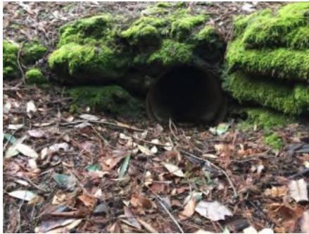
Photo 1. Culvert inlet (March 2021).
