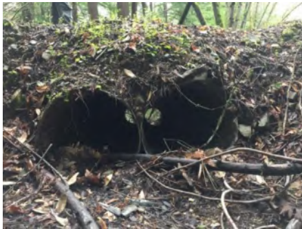
Photo 1. Culvert inlet ( March 2021 ).
