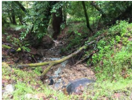
Photo 2. Culvert outlet (March 2021).
