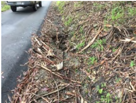
Photo 1. Culvert inlet (March 2021).
