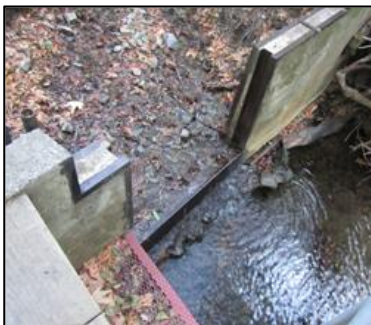
Photo 32. Flashboard weir at Hendry Intake Facility (Dec. 2013).
