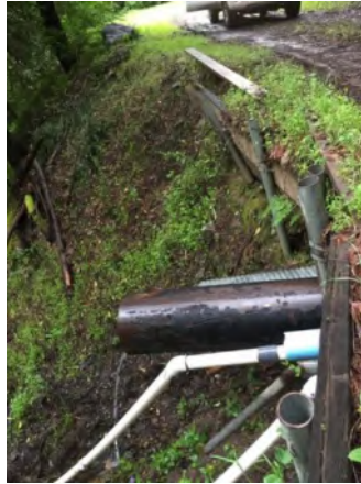
Photo 2. Culvert outlet (March 2021).
