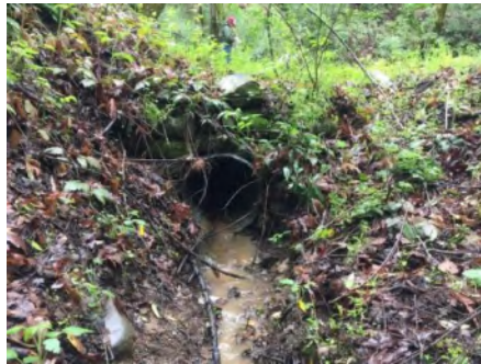
Photo 2. Culvert outlet (March 2021).
