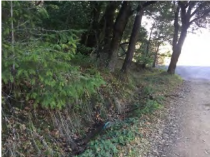
Photo 1. Culvert inlet (Jan 2019).
