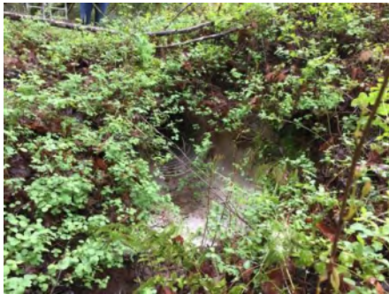
Photo 1. Culvert inlet area (March 2021).
