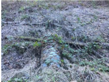
Photo 2. Culvert outlet (Jan 2019).
