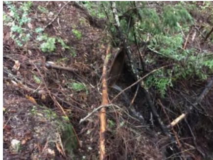
Photo 2. Culvert outlet at center (March 2021).
