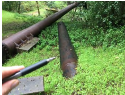
Photo 2. Culvert outlet (March 2021).
