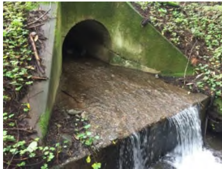
Photo 2. Culvert outlet. (March 2021).
