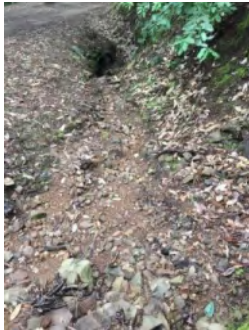
Photo 1. Culvert inlet ( March 2021 ).
