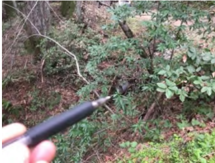
Photo 2. Culvert outlet (Jan 2019).
