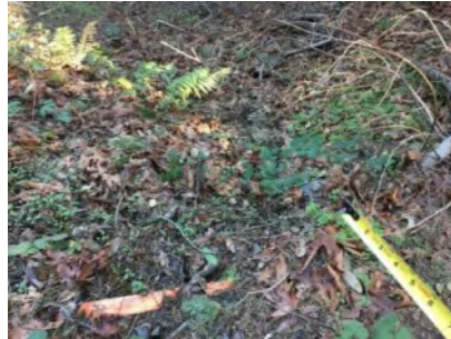
Photo 2. Culvert outlet (Jan 2019).
