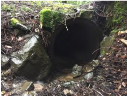
Photo 1. Culvert inlet (March 2021).
