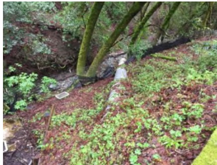
Photo 2. Culvert outlet (March 2021).
