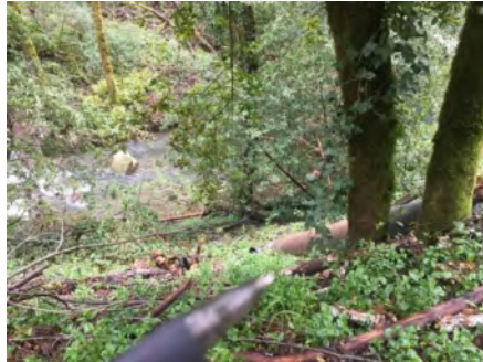
Photo 2. Culvert outlet (March 2021).
