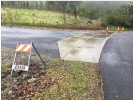
Photo 1. Culvert inlet area beneath barricade (March 2021).
