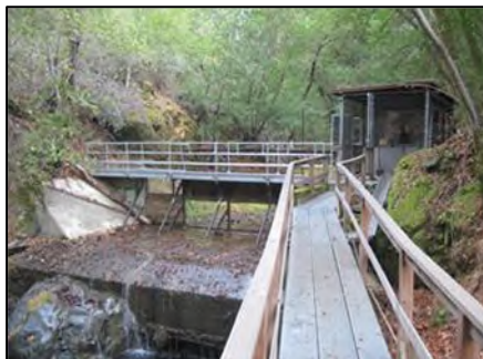
Photo 35. Lower Cavaneer Intake Facility, looking upstream (Dec. 2013).
