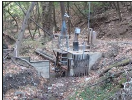
Photo 31. Hendry Intake Facility, looking downstream (Dec. 2013).
