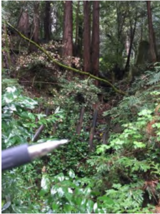
Photo 1. Culvert inlet area ( March 2021 ).
