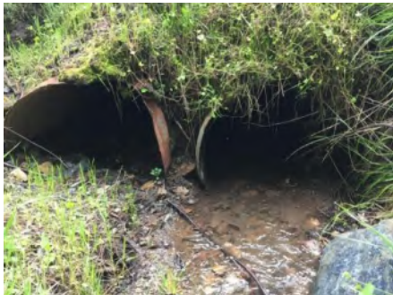
Photo 1. Culvert inlet ( March 2021 ).
