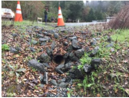
Photo 2. Culvert outlet (March 2021).
