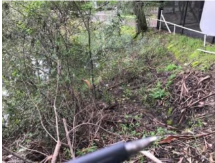
Photo 2. Culvert outlet (March 2021).
