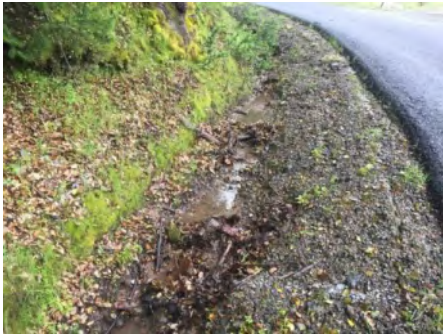
Photo 1. Culvert inlet ( March 2021 ).
