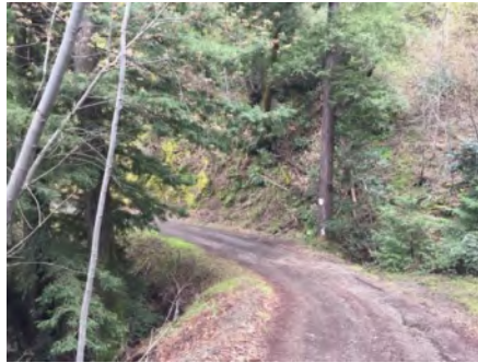
Photo 2. Culvert outlet area at left (March 2021).
