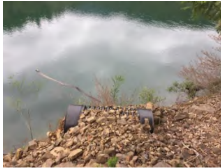
Photo 2. Culvert outlet (March 2021).
