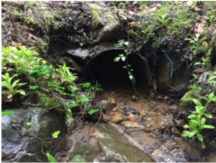
Photo 1. Culvert inlet (March 2021).
