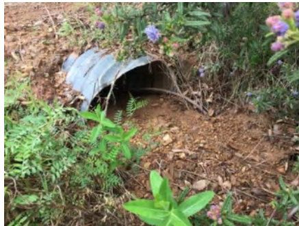
Photo 2. Culvert outlet (March 2021).
