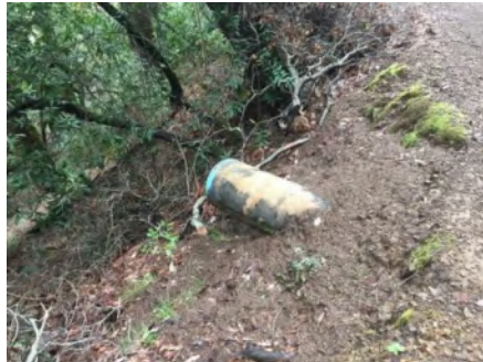
Photo 2. Culvert outlet ( March 2021 ).
