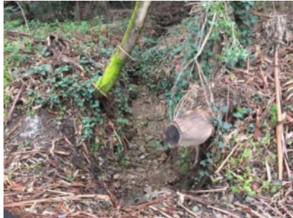
Photo 1. Culvert inlet ( March 2021 ).
