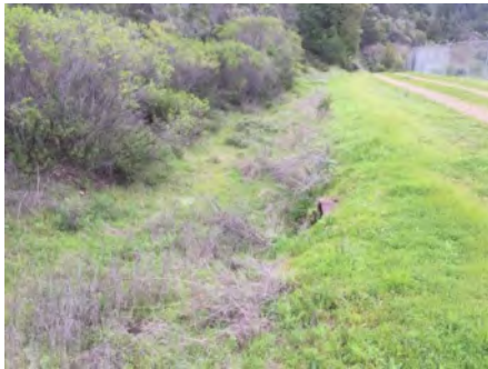
Photo 1. Culvert inlet ( March 2021 ).
