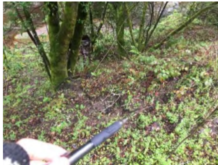
Photo 2. Culvert outlet (March 2021).
