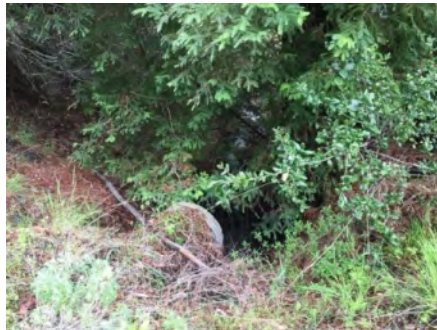
Photo 2. Culvert outlet ( March 2021 ).
