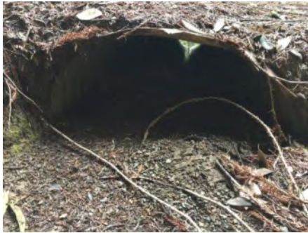
Photo 1. Culvert inlet (March 2021).
