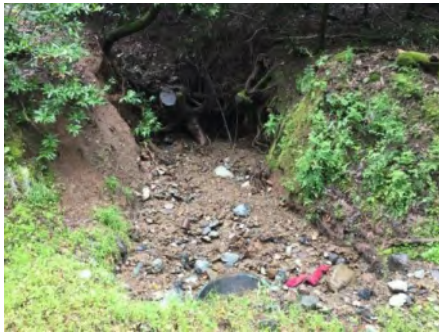
Photo 1. Culvert inlet area (March 2021).
