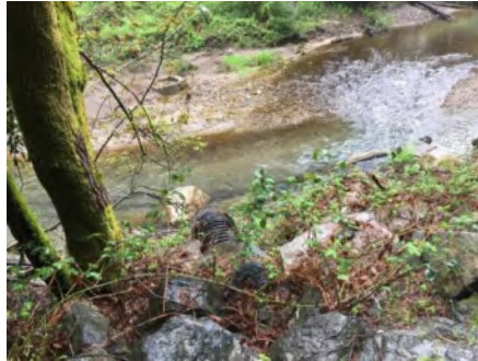
Photo 2. Culvert outlet (March 2021).
