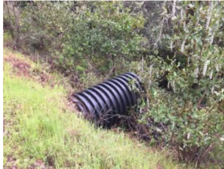
Photo 2. Culvert outlet ( March 2021 ).
