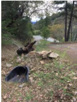
Photo 1. Culvert inlet ( March 2021 ).
