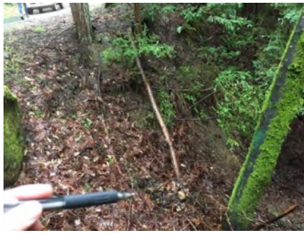
Photo 2. Culvert outlet ( March 2021 ).
