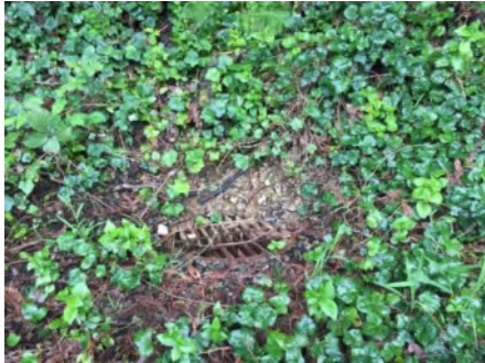
Photo 1. Culvert inlet area (March 2021).
