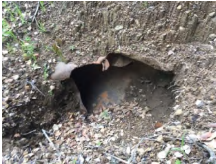
Photo 1. Culvert inlet ( March 2021 ).
