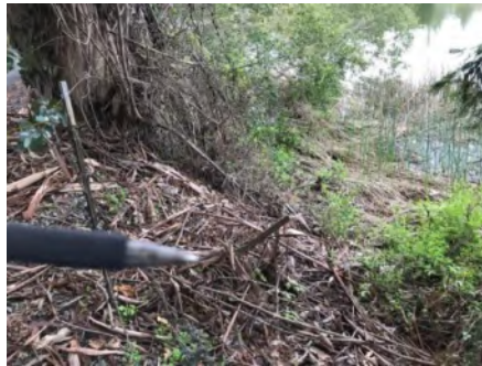
Photo 2. Culvert outlet (March 2021).
