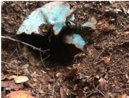
Photo 1. Culvert inlet ( March 2021 ).
