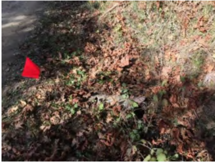
Photo 1. Culvert inlet area (Jan 2019).
