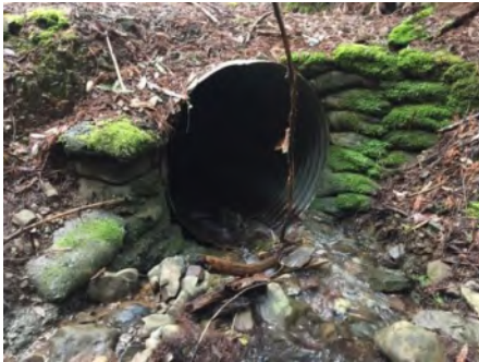
Photo 1. Culvert inlet (March 2021) .
