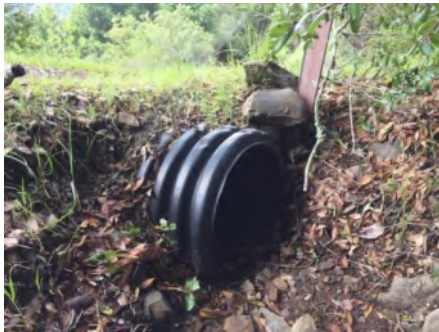
Photo 1. Culvert inlet ( March 2021 ).
