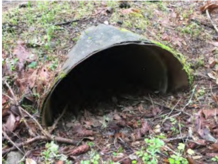
Photo 1. Culvert inlet (March 2021).
