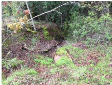
Photo 2. Culvert outlet ( March 2021 ).
