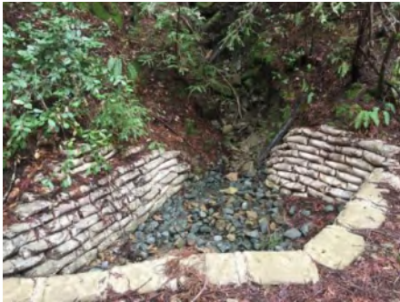
Photo 1. Culvert inlet area (March 2021).
