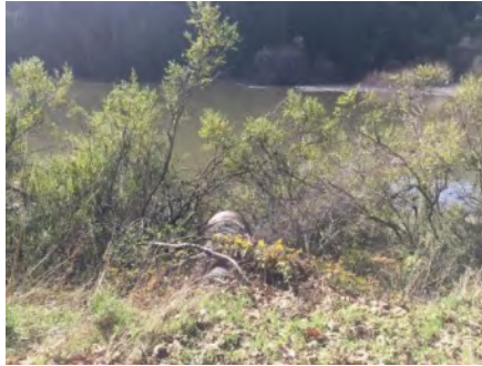
Photo 2. Culvert outlet area (Jan 2019).
