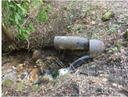
Photo 2. Steep bank on the eastern side of John Nicholas Trail (Jan 2019).
