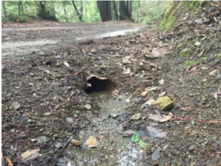
Photo 1. Culvert inlet ( March 2021 ).
