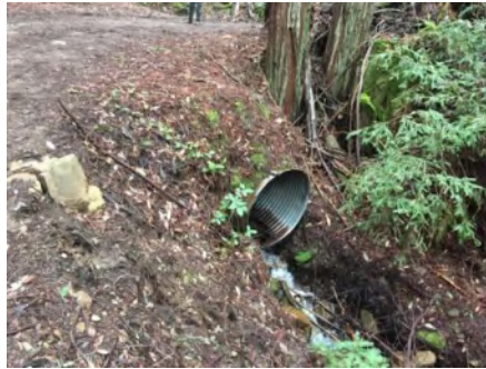
Photo 2. Culvert outlet area (March 2021) .
