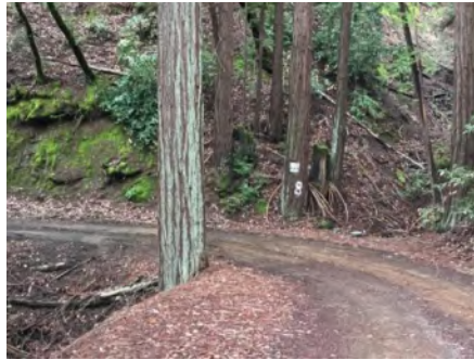
Photo 2. Culvert outlet area at left (March 2021).
