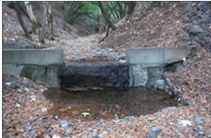
Photo 44. Trout Creek Intake Facility weir and downstream pool (Oct. 2013).
