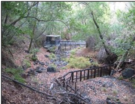
Photo 38. Debris rack in near ground to right, Lower Cavaneer Intake Facility in background (Dec. 2013).
