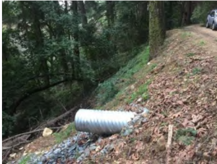
Photo 2. Culvert outlet (Jan 2019).
