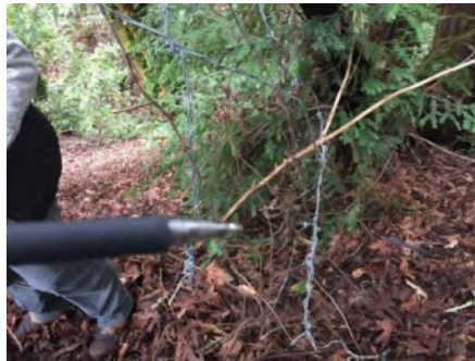
Photo 2. Culvert outlet area ( March 2021 ).
