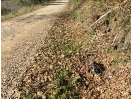
Photo 1. Culvert inlet area (Jan 2019).
