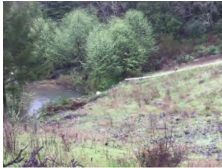
Photo 2. Potential culvert outlet area (March 2021).
