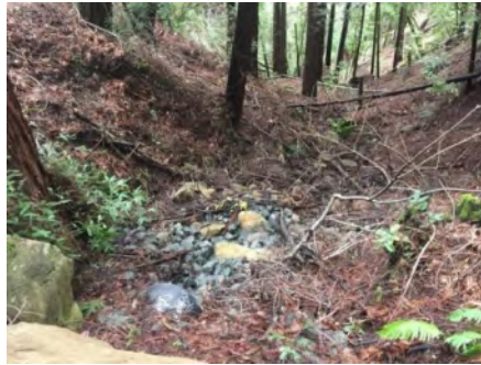
Photo 2. Culvert outlet (March 2021).
