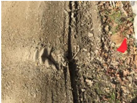
Photo 1. Culvert inlet area (Jan 2019).
