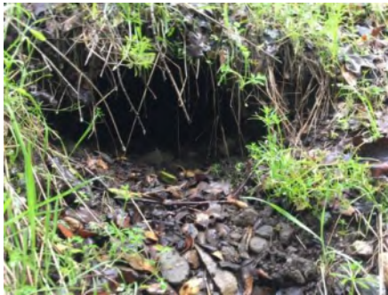
Photo 2. Culvert outlet ( March 2021 ).
