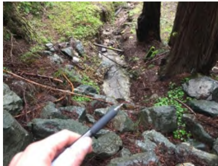
Photo 2. Culvert outlet (March 2021).
