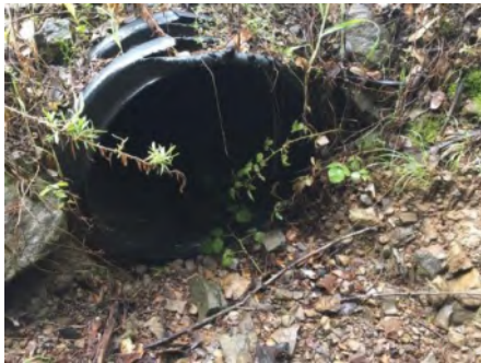
Photo 1. Culvert inlet ( March 2021 ).
