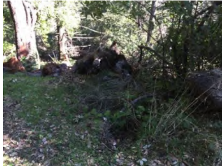
Photo 2. Culvert outlet (Jan 2019).
