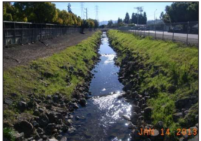
Photo 6. Sunnyvale East Channel at Station 156+28.
