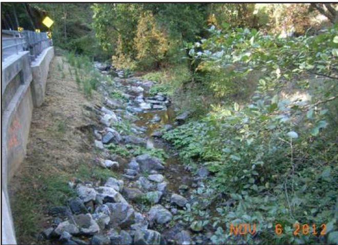
Photo 3. Stevens Creek at Station 931+46.
