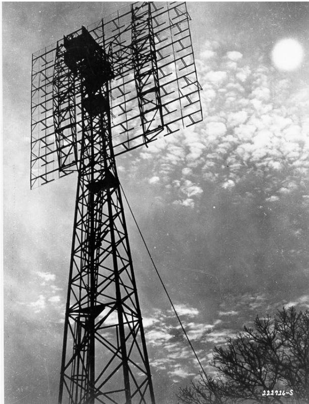
Project Diana, 1946 - Radar installation at Fort Monmouth, New Jersey, juxtaposed against the moonlight sky to illustrate the accomplishment of bouncing communication signals through space. (Photo from Signal Historical Collection)
