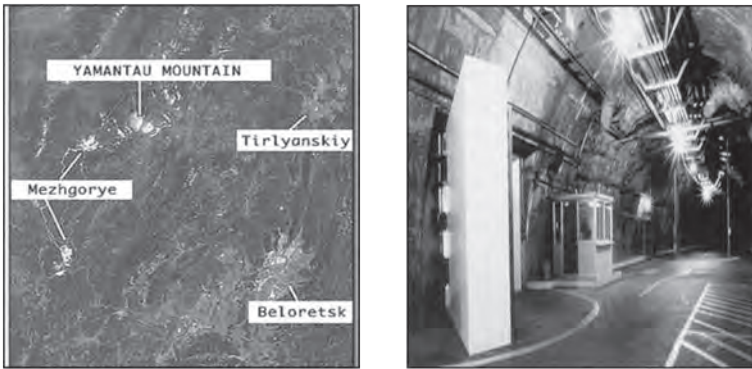
Figure 1-7. Russian Underground Nuclear Complex at Yamantau.
