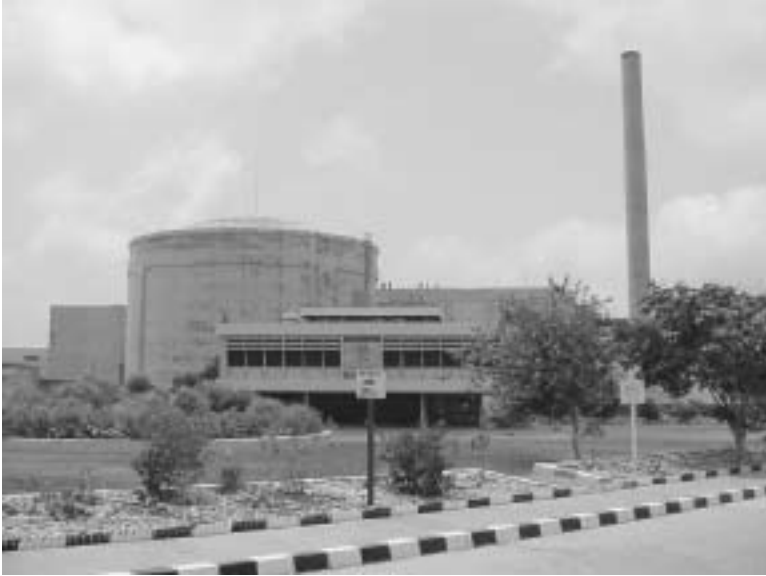
Figure 1. The Karachi Nuclear Power Plant (KANUPP).
