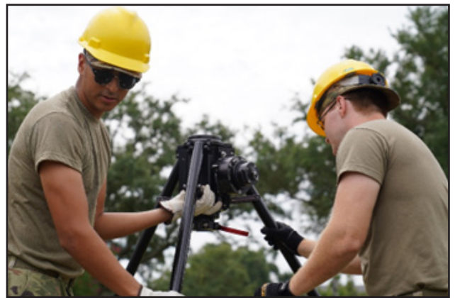
U.S. Air Force Airman Francisco Rebolledo and Airman 1st Class James Miller, 338th Training Squadron Radio Frequency Transmission Systems students, practice building a Blue Sky antenna mast during class at Keesler Air Force Base, Mississippi, Sept. 6, 2022. The 338th TRS specializes in two pipeline courses, RF Transmissions Systems and Network Operations. (U.S. Air Force photo by Airman 1st Class Elizabeth Davis)
