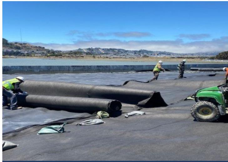
Drainage geocomposite (left) and high-density polyethylene (HDPE) (right) were installed over the site to drain excess water in cover soils (wetlands excepted)
