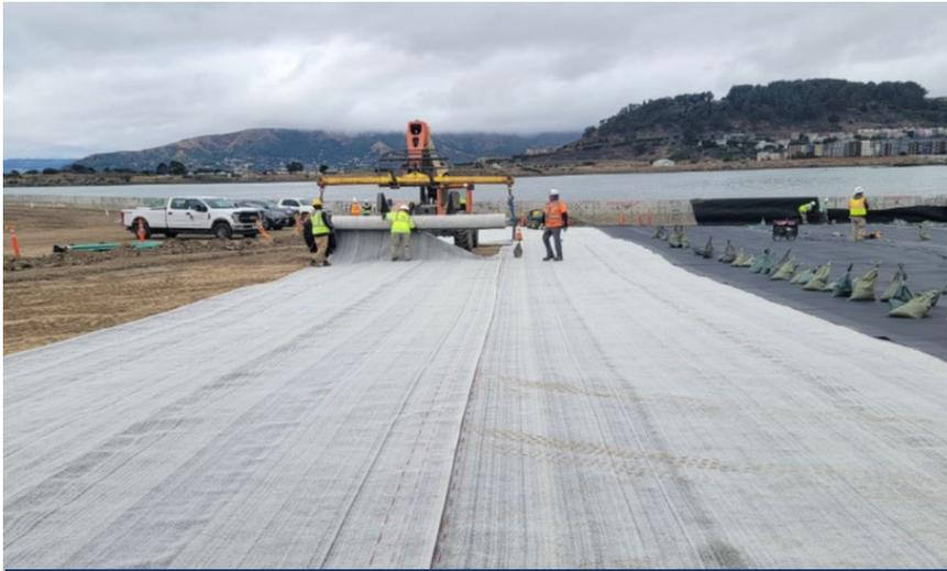
A geosynthetic clay liner (GCL) was installed for extra protection over landfill wastes
