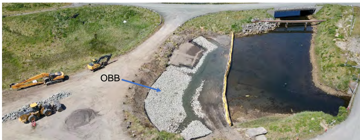
Photo of Oleophilic Bio-Barrier during construction on July 11, 2022
